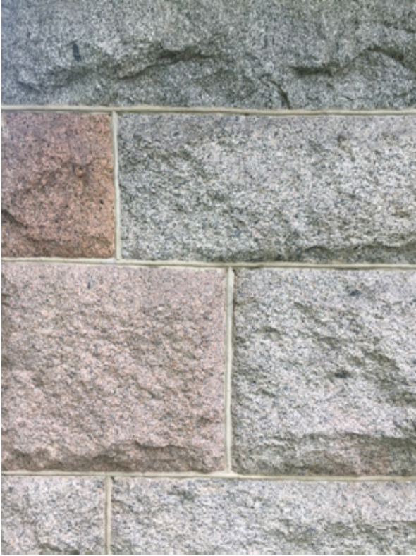
Figure 8. The reddish and greyish Kalvola granite on the façade of the Kalvola Church. Photo: Olavi Selonen.
