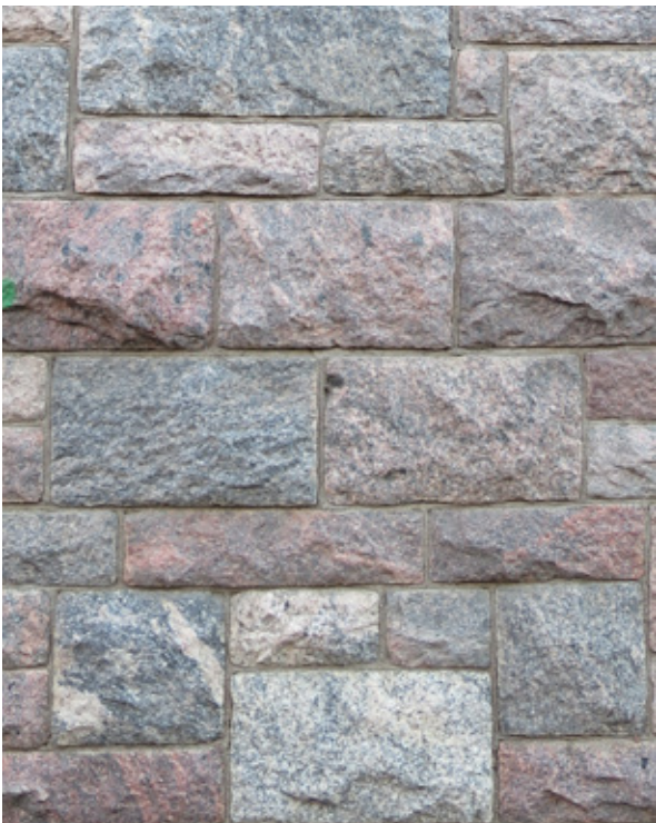
Figure 5. Various appearances of the Helsinki granite on the lower façade of the Falken building. Photo: Olavi Selonen.
