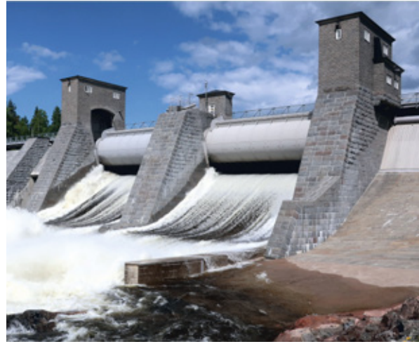
Figure 2. Structures of the Imatra power plant in southeastern Finland are covered with the Antrea granite. Photo: Paavo Härmä.
