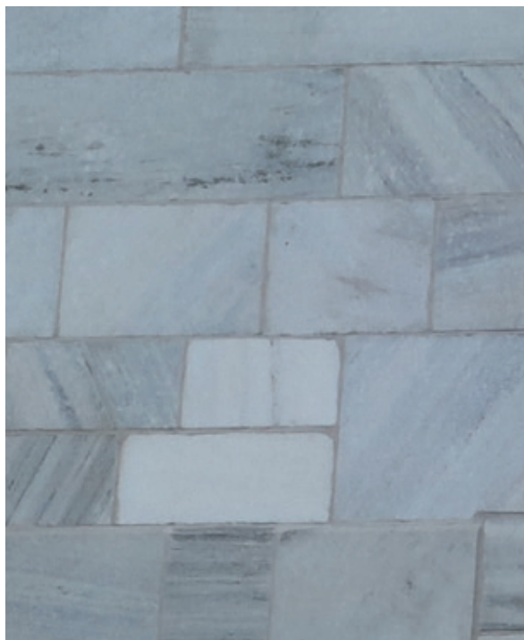
Figure 28. Various appearances of the Förby marble on the façade of the Marble Palace in Helsinki. Photo: Paavo Härmä.
