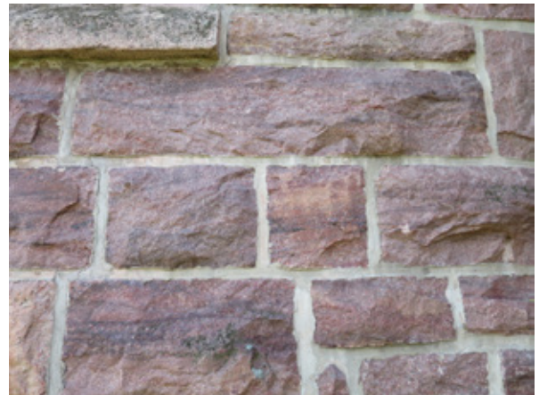
Figure 32. The Satakunta sandstone on the facade of the Luvia Church. Photo: Olavi Selonen.
