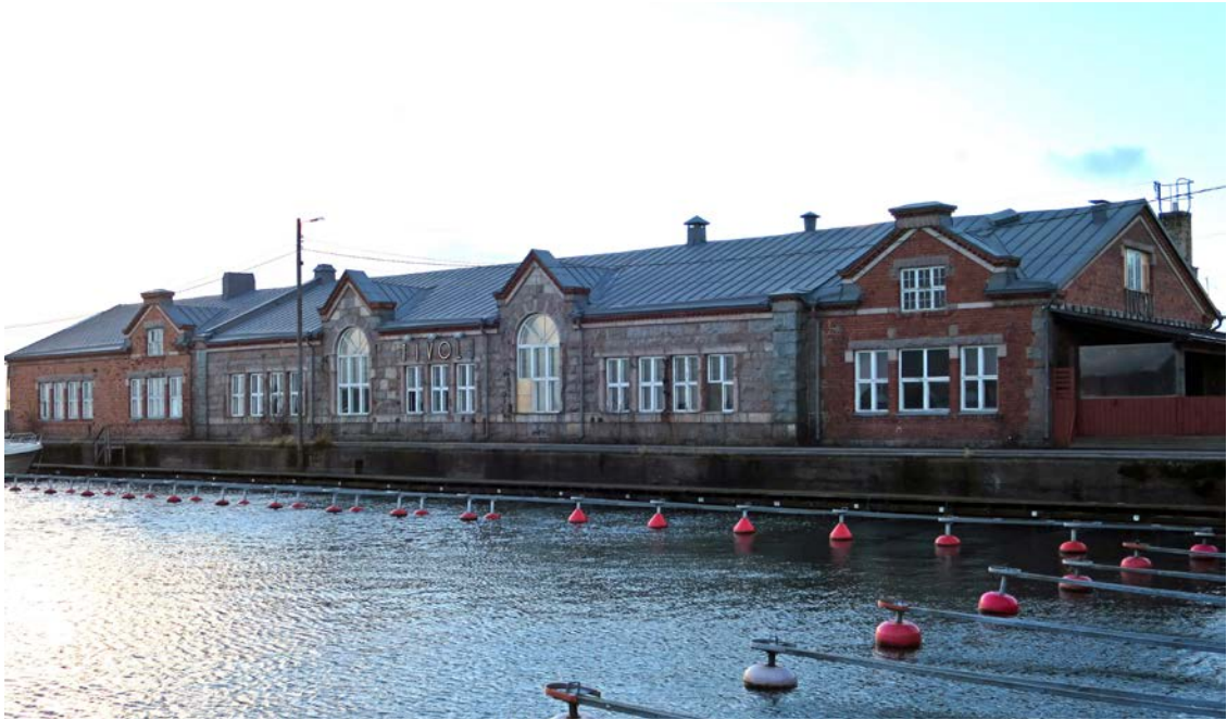
Figure 1. The former processing plant building of the Ab Granit company, Hanko (1896). Hanko granite. Photo: Olavi Selonen.
