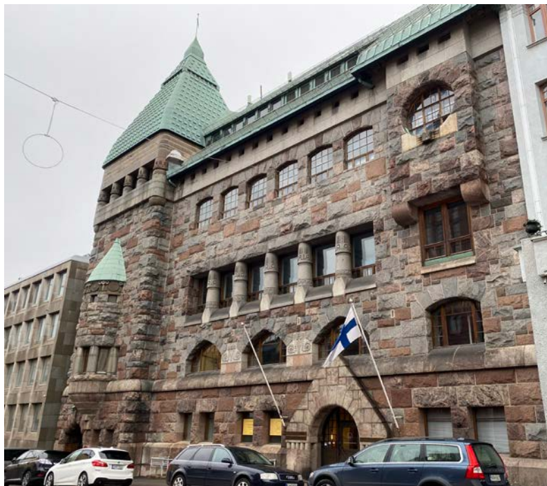
Figure 5. The Helsinki Telephone Company building (1905), Helsinki. Uusikaupunki granite, local granite, local gneiss. Photo: Olavi Selonen.
