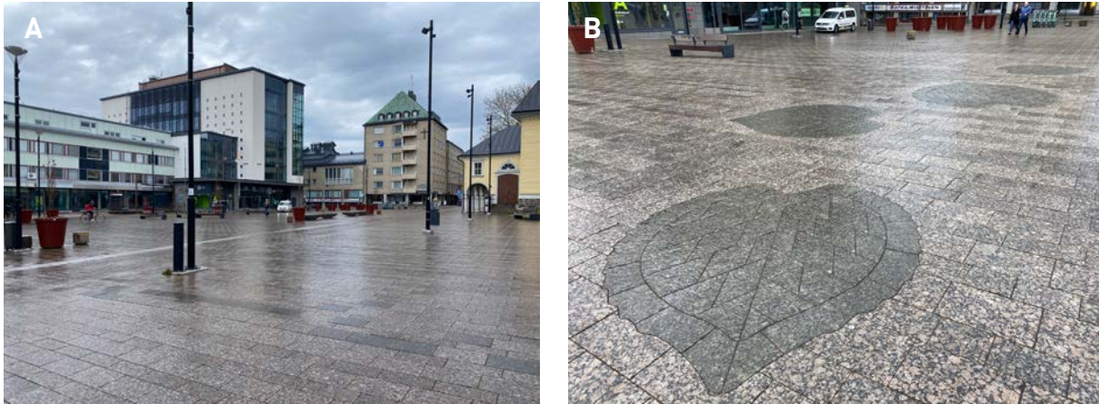
Figure 13. The paving of the Maria Square is realized in slabs of brown rapakivi granite from Ylämaa ( Baltic Brown ) (A), while the linden leaves pointing in intercardinal compass directions are made of green rapakivi granite from Ylämaa ( Baltic Green ) (B). Photos: Olavi Selonen.
