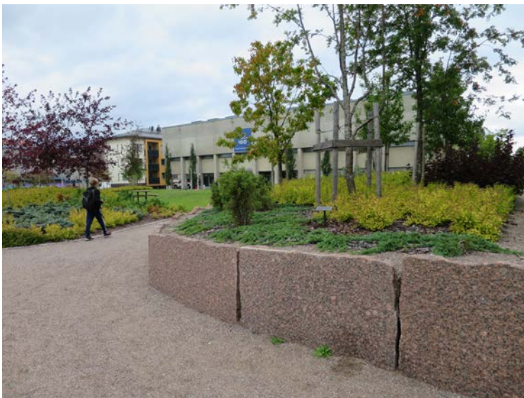
Figure 12. Cheek stones from a local stone processing factory are applied as walls in the Paasikivenpuisto Park. The surface has a flamed finish. Photo: Olavi Selonen.
