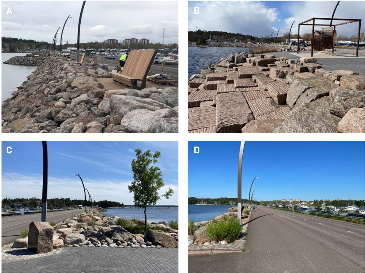
Figure 1. Juha Vainion katu street. A. View to the west in 7.5.2019. B. View to the west in 29.4.2021. C. View to the east in 29.6.2021. D. View to the west in 16.7.2025. See also map in Fig. 3. Photos: Olavi Selonen.
