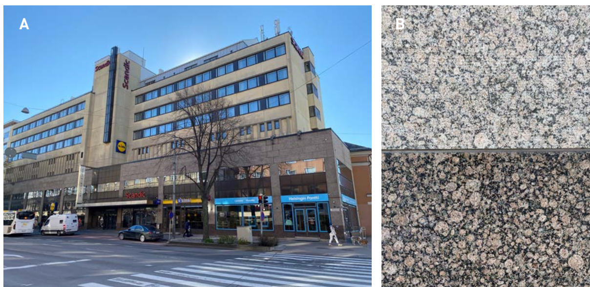
Figure 19. The lower façade of the hotel building at No 4 Eerikinkatu Street is faced with slabs of brown rapakivi granite from Ylämaa ( Baltic Brown ) (A) with bush hammered and polished finish (B). The different effects of the surface treatments on the appearance of the stone can be clearly seen here as the bush hammered (B, upper) slabs are visibly lighter in colour compared to the polished ones (B, lower). Fine processing (e.g. polishing) produces glossy surfaces showing the natural patterns, colours, and textures of a rock. Coarse finishing (e.g. bush hammering) leads to a different effect: the stone appears lighter but its pattern becomes indistinct, and the original tint disappears. Photos: Olavi Selonen.
