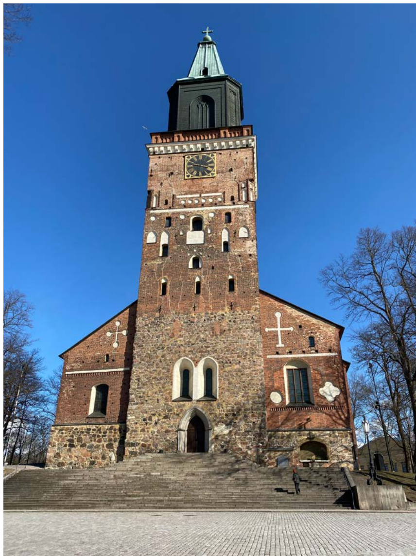
Figure 2. A mixture of local rock types of varying shapes is used in construction of the foundation of the Turku Cathedral. Photo: Olavi Selonen.
