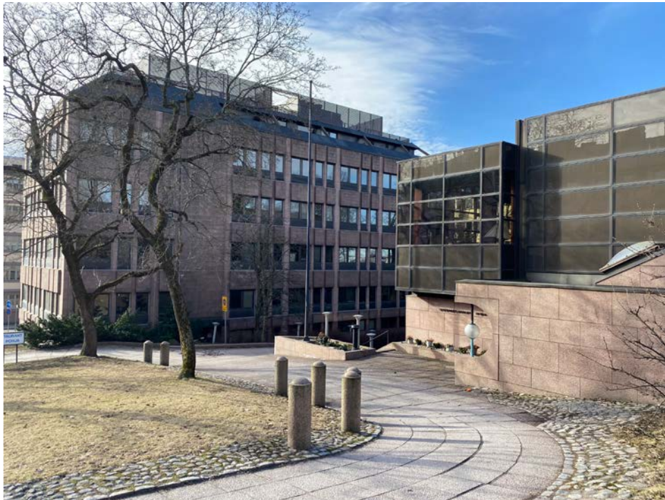
Figure 14. The Suomalainen Pohja restaurant building (in the foreground) and the Sampo office building (in the background) are clad with flamed slabs of red rapakivi granite from Taivassalo ( Balmoral Red cg ). Photo: Olavi Selonen.
