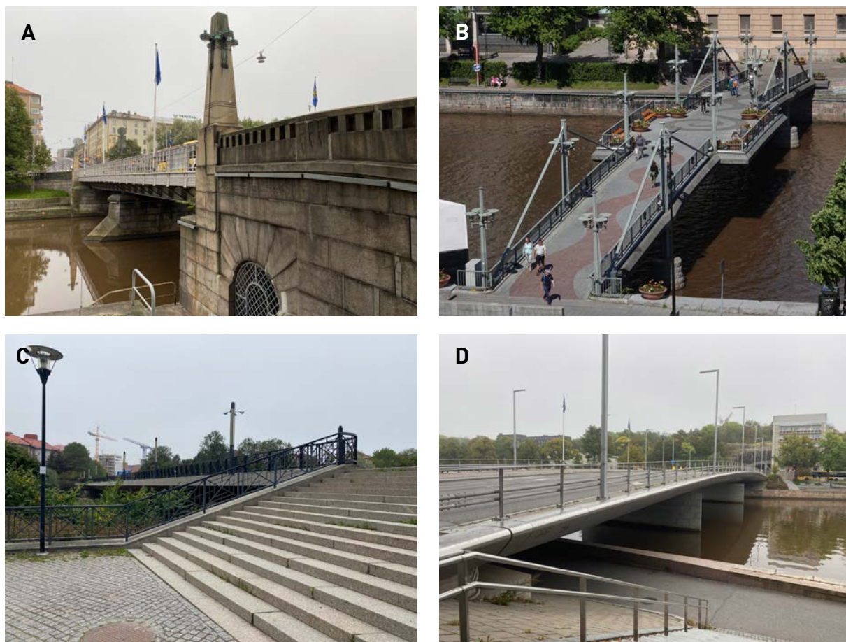
Figure 26. A. Local grey granite from Turku is applied in the constructions of the Auransilta Bridge. B. The deck of the Teatterisilta Bridge is covered with Kuru Grey , Amadeus , Baltic Green , Carmen Red granites. C. All stone constructions of the Tuomaansilta Bridge are made in brown rapakivi granite from Taivassalo ( Esko Brown ). D. The pillars of the Myllysilta Bridge are faced with grey granite from Kuru ( Kuru Grey ). The stairs, benches, and paving at both ends of the bridge are made in the same granite. Photos A, C, D: Olavi Selonen, B: Carl Ehlers.
