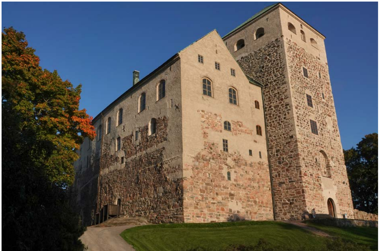
Figure 1. A mixture of local rock types are used in construction of the Turku Castle. Local rounded boulders abound in the walls. Photo: Carl Ehlers.
