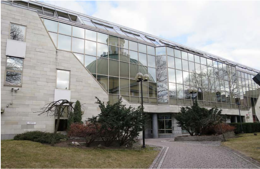
Figure 15. The Aleksandra office building is faced with slabs of Lokka Quartzite from northern Finland with a split finish. Photo: Olavi Selonen.
