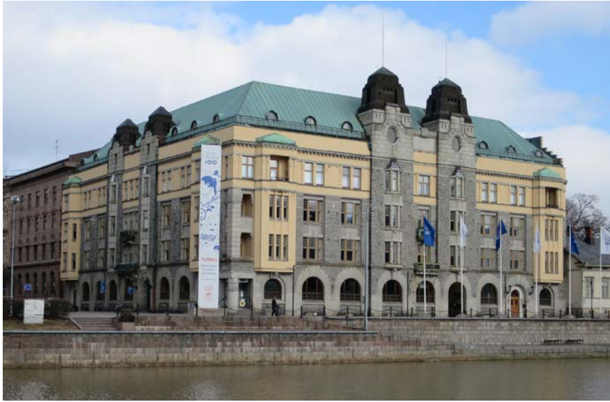
Figure 7. The façade of the Fire Insurance Company building is partly made of rock-faced and pointed light grey granite (trondhemite) from Uusikaupunki ( Birkhall Grey/Glencoe Grey ). Photo: Olavi Selonen.
