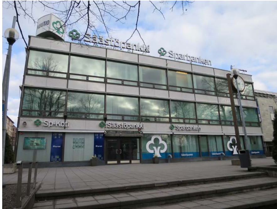
Figure 12. The Salama House was originally clad with white Italian Carrara Marble, but because of bending of the marble slabs, the facing was replaced with polished Norwegian granite (trondhjemite) ( Støren ) at the beginning the 2000s. Photo: Olavi Selonen.
