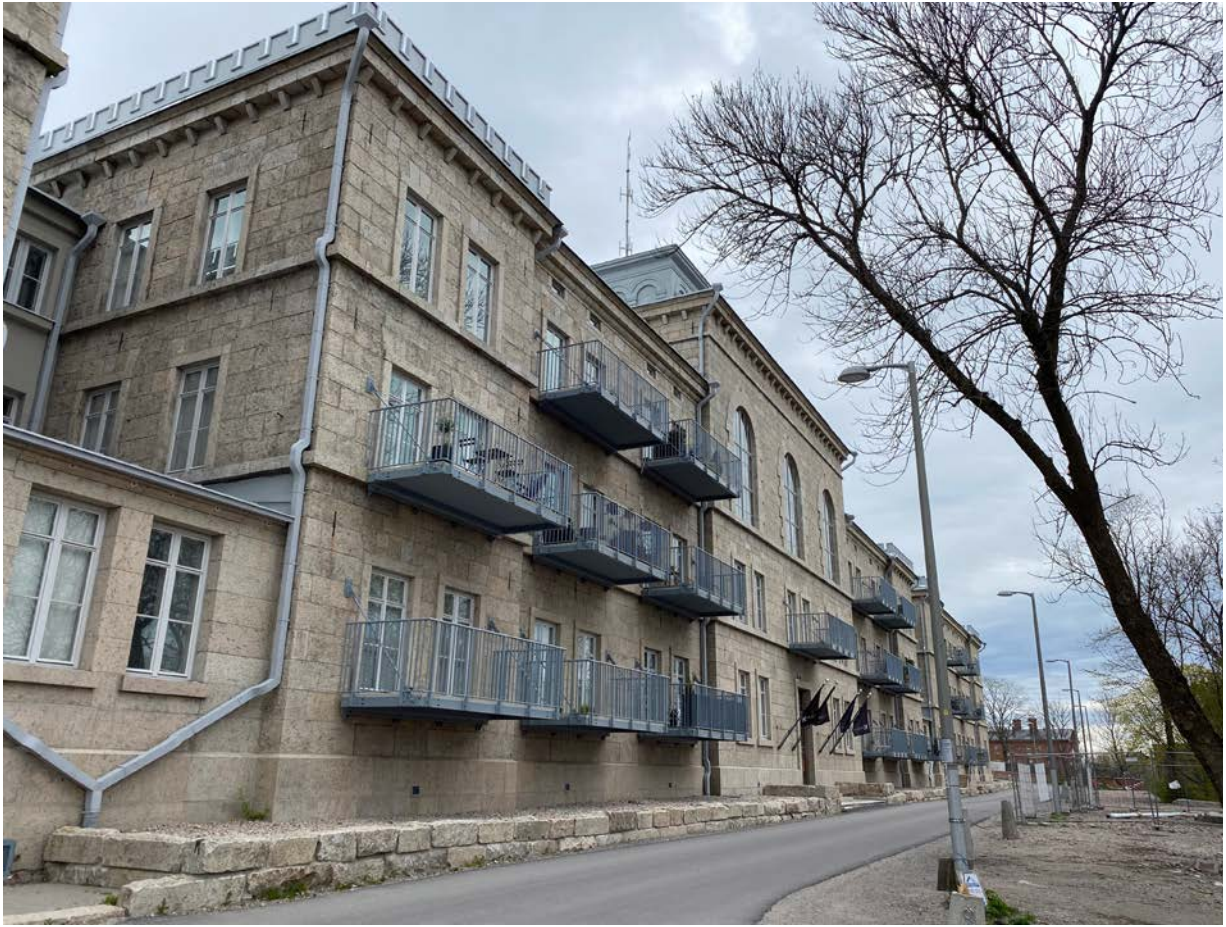
Figure 5. The façade of the former Central Prison of Kakola is made of blocks of grey local granite quarried from the construction site. Photo: Olavi Selonen.
