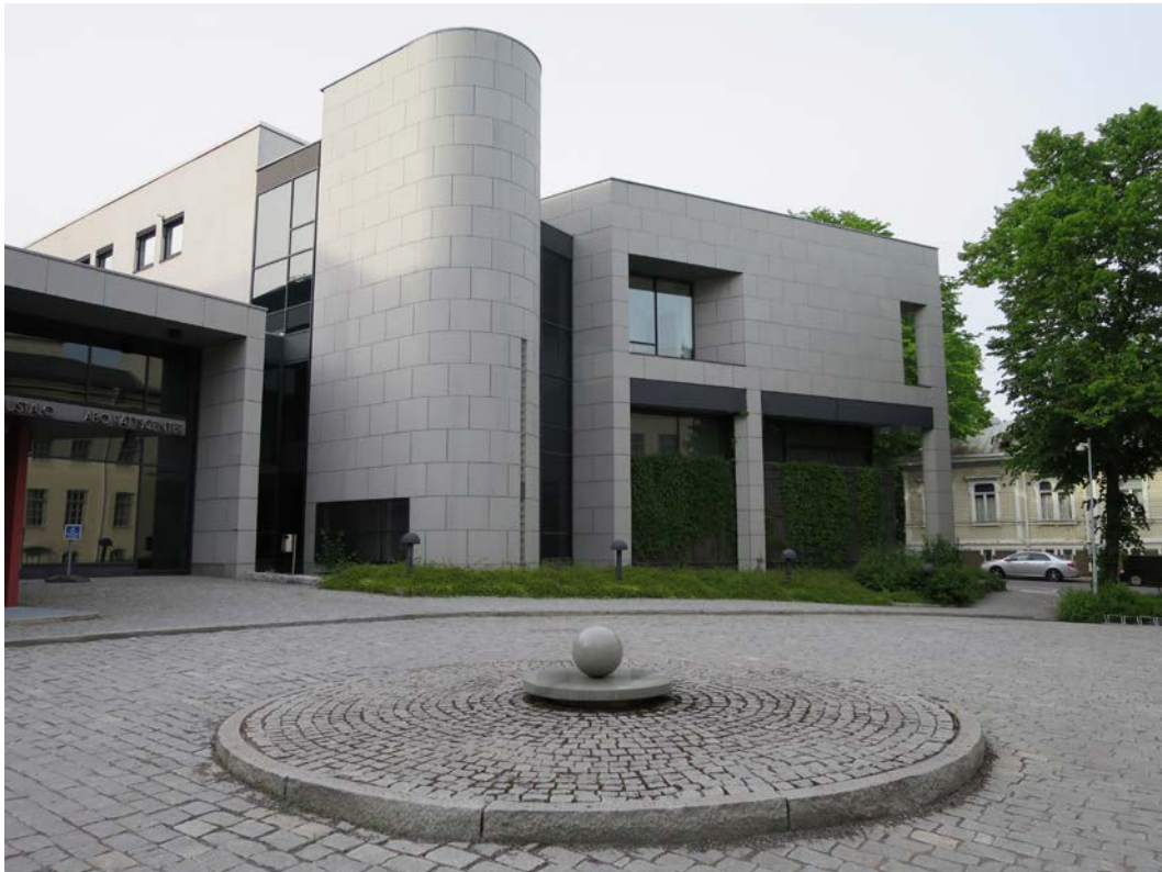
Figure 16. The Turku Courthouse building is clad with grey granite from Kuru ( Kuru Grey ) with a flamed finish. The application gained the “Great Stone Prize” of the Finnish Natural Stone Association in 1998 for the successful use of natural stone in construction. Photo: Olavi Selonen.
