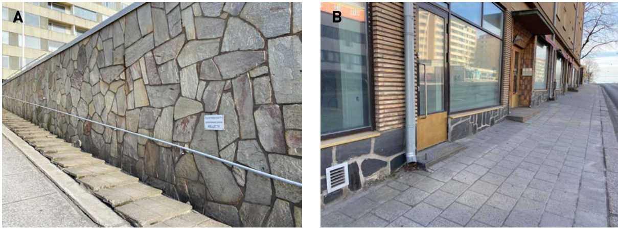
Figure 11. Light schist is applied as facing at No 8–12 Uudenmaankatu Street (A) while dark schist can be seen in the plinth of the building at No 13 Uudenmaankatu Street (B). Photos: Olavi Selonen.
