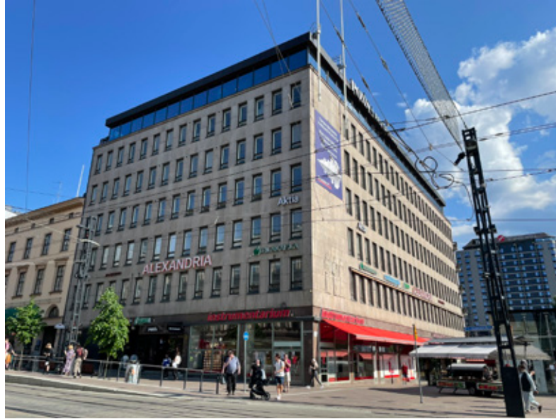
Figure 7. The upper part of the Bank of Finland building (1943) is faced with red medium-grained porphyritic Kuru granite, while the lower façade is realized in red granite from Kökar. Photo: Olavi Selonen.
