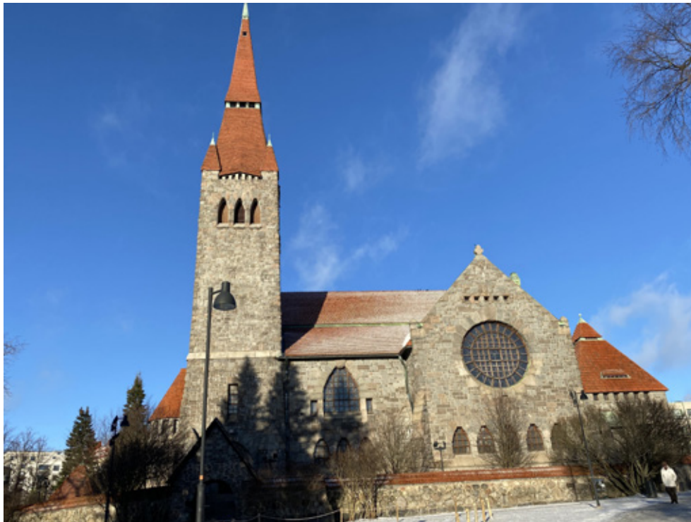
Figure 2. The façade of the Tampere Cathedral (1907) is constructed from grey Uusikaupunki and Kuru granites and from other rock-faced even-grained granitic rocks. Reddish rock-faced coarse-grained porphyritic Kuru granite is also applied in the façade. Photo: Olavi Selonen.
