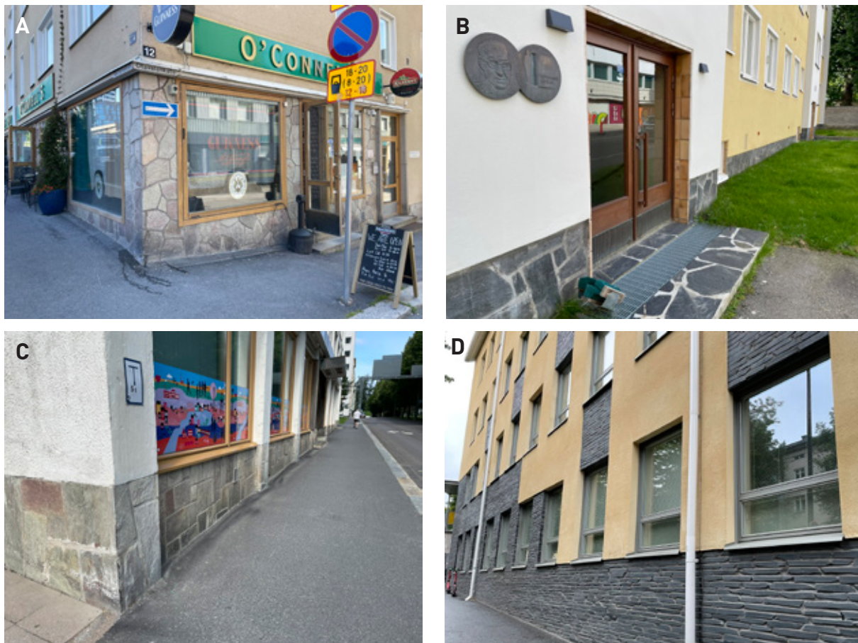
Figure 8. Use of schists in Tampere. A. No. 24 Rautatiekatu Street (1957), light schist. B. The Amurinlinna Block (1949–1955): No. 15 Puuvillatehtaankatu Street, dark schist. C. The Amurinlinna Block (1949–1955): No. 12 Hämeenpuisto Street, light schist. D. The Tampere International School (2017), dark schist masonry. See text for explanation. Photos: Olavi Selonen.
