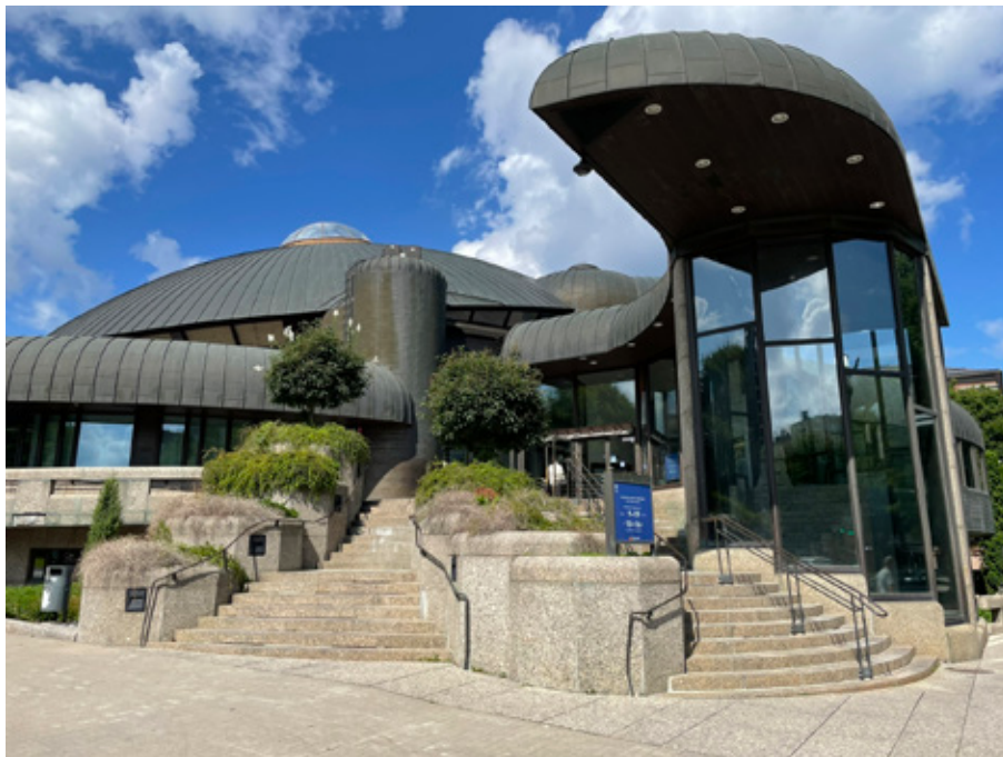
Figure 9. Part of the façade, stairs, and masonry of the Tampere City Library Metso (1986) are constructed from brown rapakivi granite from Ylämaa ( Baltic Brown ). Photo: Olavi Selonen.
