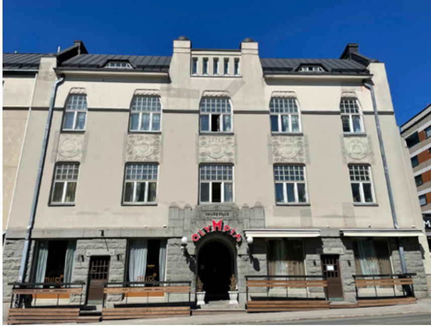
Figure 4. The lower façade, the foundation, and the portal of the house of the Tampere Association for workers working outside (1908) are made in grey Kalvola granite. Photo: Olavi Selonen.
