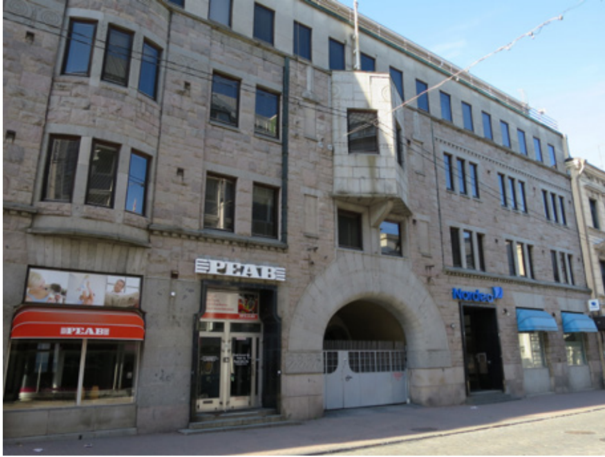
Figure 3. The upper façade the Tampere KOP bank building (1907) is realized in reddish Kalvola granite, while the lower and middle parts are made in greyish Kalvola granite. Photo: Olavi Selonen.
