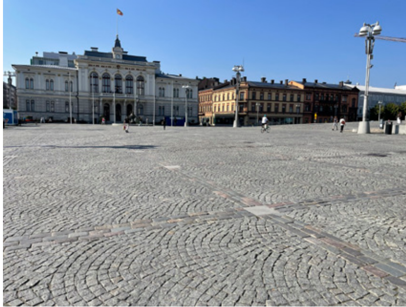
Figure 11. The paving of the Tampere Central Square is constructed from setts and cubes of grey Kuru granite. In addition, cobblestone is applied. Photo: Olavi Selonen.
