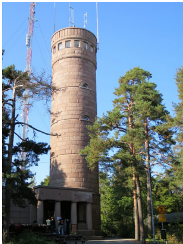
Figure 22. The façade of the Pynnikki Observation Tower (1929) is made in red rapakivi granite from Vehmaa ( Balmoral Red fg ). Photo: Olavi Selonen.
