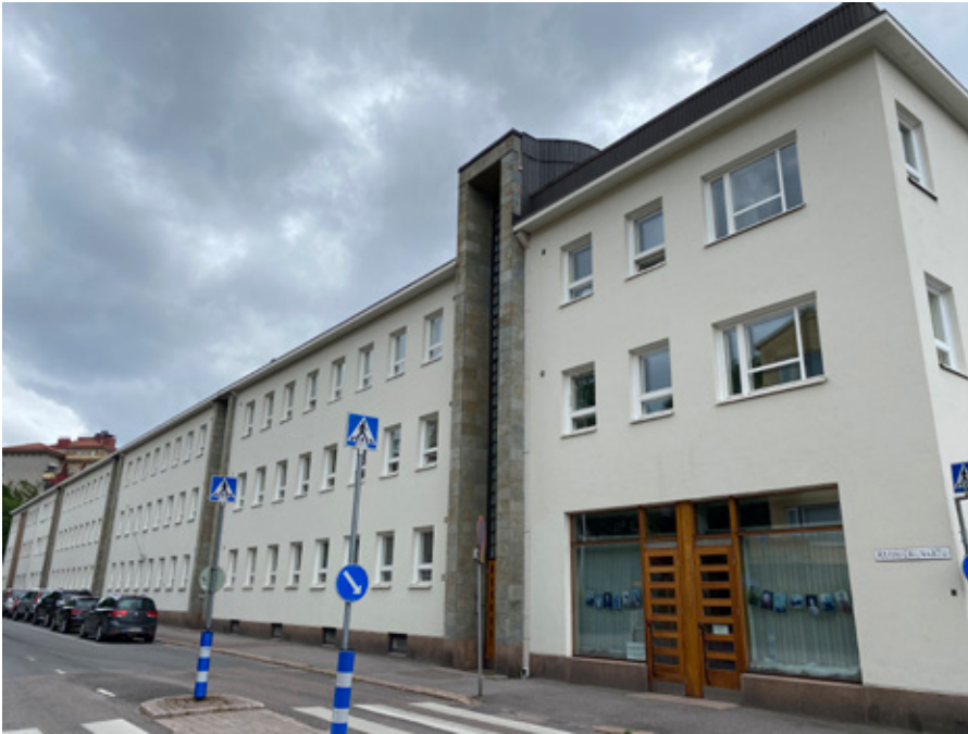
Figure 9. The high portals of the apartment house (1941) at No 35 Kariniemenkatu Street are made in soapstone from Nunnanlahti, Juuka of eastern Finland. Photo: Olavi Selonen.
