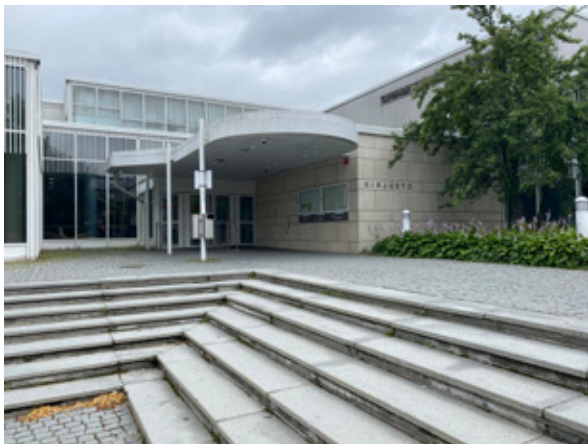
Figure 3. The Lahti City Library building is partly clad with travertine from Rome, Italy ( Travertino Romano ). The paving and the stairs in front of the building are made in grey granite from Kuru ( Kuru Grey ). Photo: Olavi Selonen.
