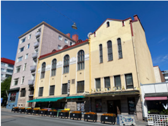
Figure 1. The portal and the foundation of the House of Lahti Printing and Newspaper Ltd (currently the Pikkuaterin House) are made in red rapakivi granite from Myrskylä ( Rayham Red/Mahogany Red ). Photo: Olavi Selonen.
