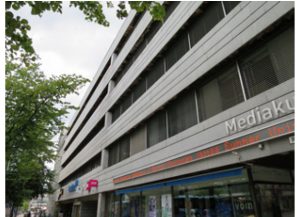
Figure 2. The façade of the extension to the Lahti KOP bank building is faced with grey Uusikaupunki granite (trondhjemite) ( Birkhall Grey/Glencoe Grey ). Photo: Olavi Selonen.
