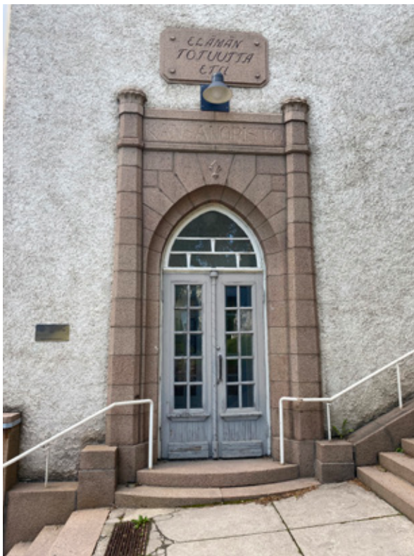
Figure 2. The portal of the Lahden Kansanopisto school building. Red Myrskylä granite. Photo: Olavi Selonen.
