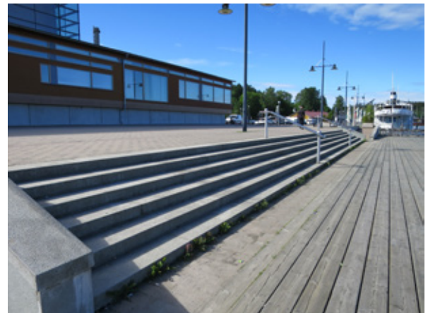
Figure 4. The stairs at the backside of the Sibelius Hall are made in grey granite from Kuru ( Kuru Grey ). Photo: Olavi Selonen.
