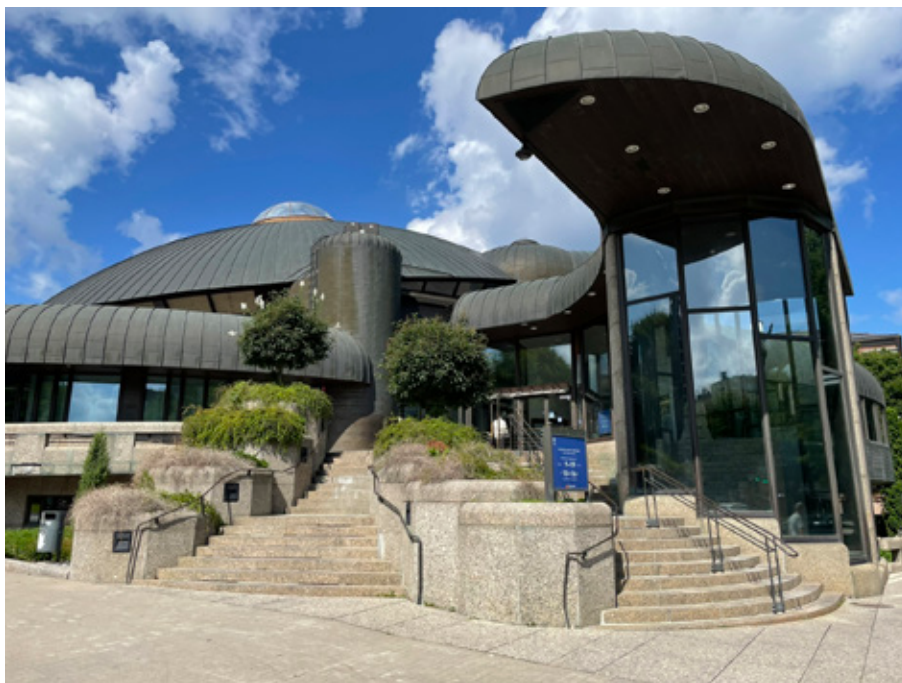
Figure 9. Part of the façade, stairs, and masonry of the Tampere City Library Metso (1986) are constructed from brown rapakivi granite from Ylämaa ( Baltic Brown ). Photo: Olavi Selonen.
