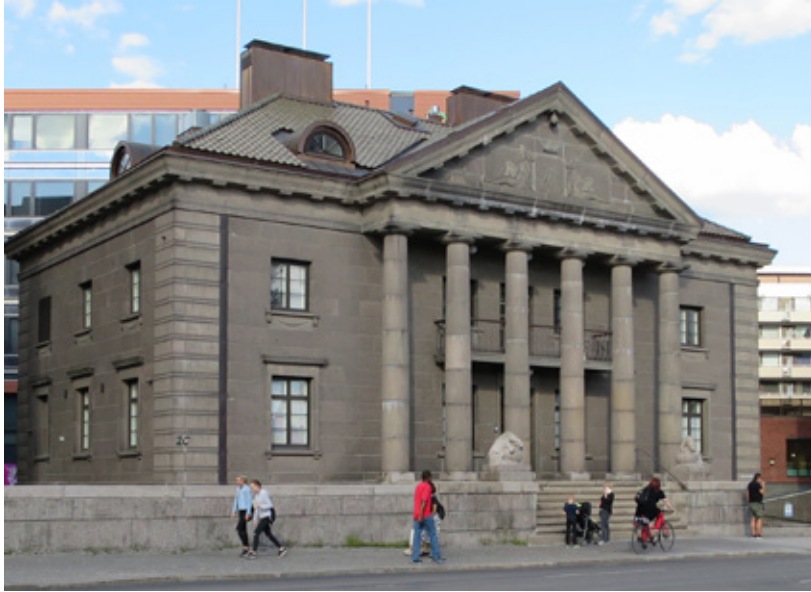
Figure 6. The Haarla Palace (1923) is clad with red medium-grained porphyritic Kuru granite. Photo: Olavi Selonen.
