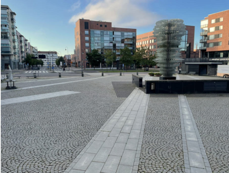
Figure 16. The grey granite from Kuru ( Kuru Grey ) has been extensively used at the Pellavantori Square as slabs, setts, cubes, stairs, and façade material. Photo: Olavi Selonen.
