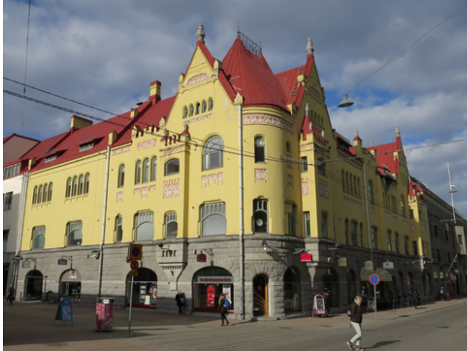
Figure 1. The lower façade and the plinth of the Tirkkonen Commercial House (1901) are made in grey Kuru granite. Photo: Olavi Selonen.
