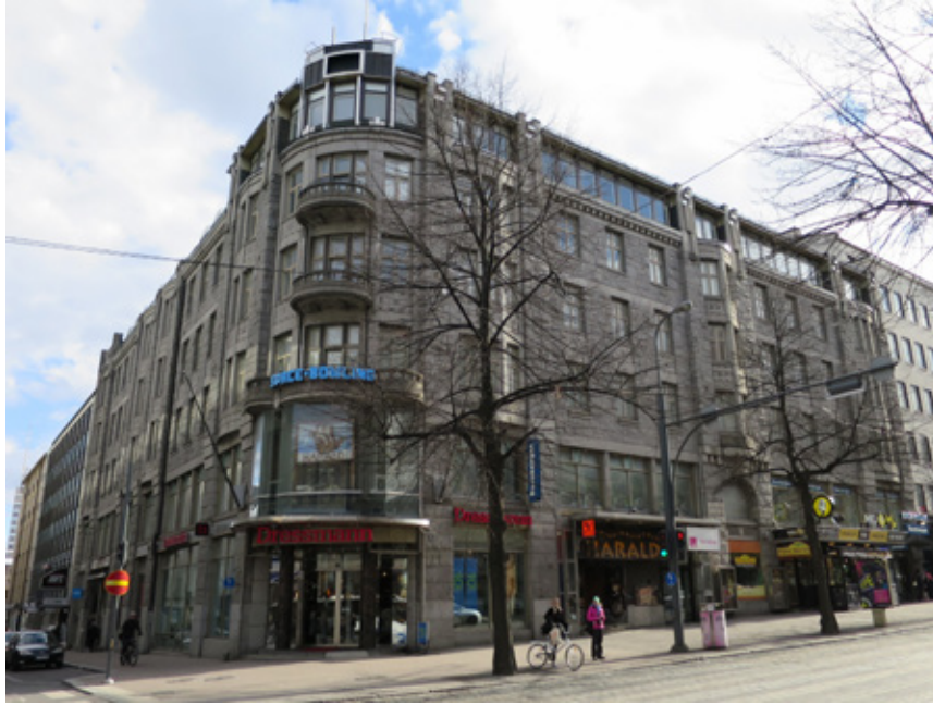
Figure 5. The façade of the Oтра Oy Commercial House (1914) is constructed from grey Kuru granite. Photo: Olavi Selonen.
