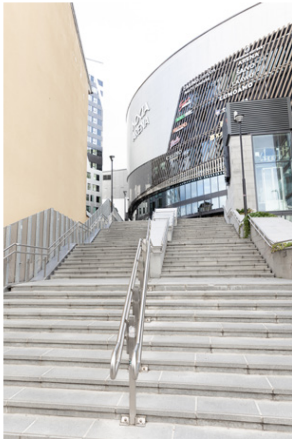
Figure 10. The stairs from the main entrance of the Tampere Deck Arena (2021) down to the Sorinkatu Street are made in grey granite from Kuru ( Kuru Grey ). Photo: Tampereen Kovakivi Oy.
