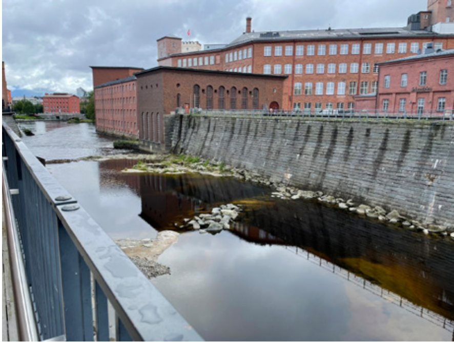
Figure 13. The embankments of the Tammerkoski Rapids are constructed from blocks of grey Kuru granite. Photo: Olavi Selonen.
