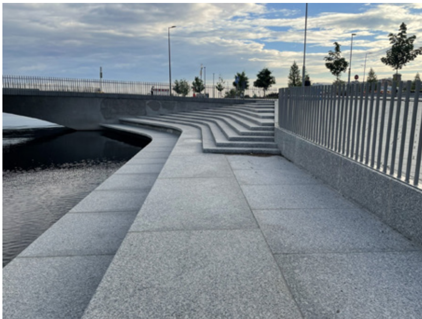
Figure 17. The paving, stairs, embankment, walls, masonry, and planting pools at the Gustaf Aspin aukio Square (2023) are done in light grey/yellowish granite from Viitasaari ( Viitasaari Light ). Photo: Olavi Selonen.
