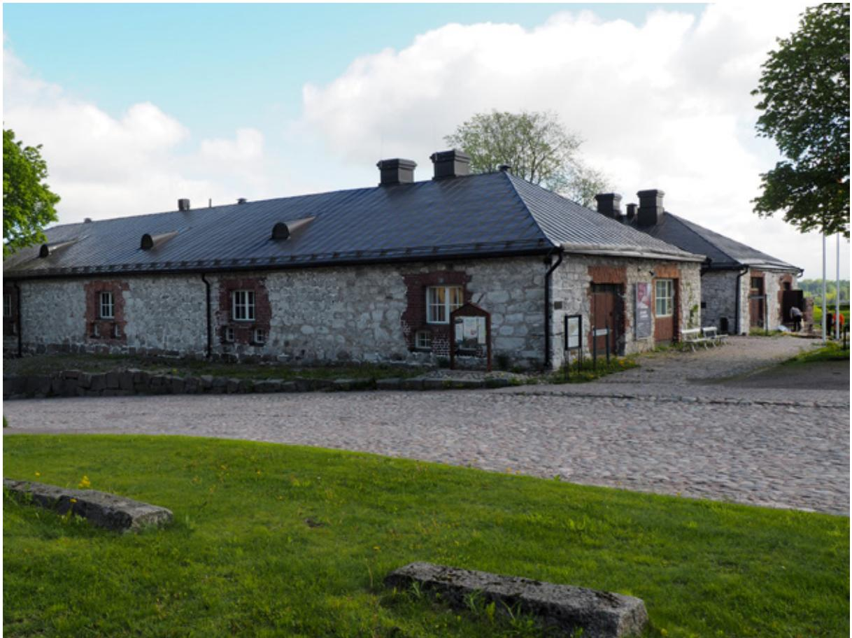
**Figure 2.** The South Karelia Museum. Blocks of local hard granitic rock types are applied in the lower parts of the buildings and blocks of limestone from the local Ihalaisten quarry in the upper parts. Photo: Heidi Laxström.
