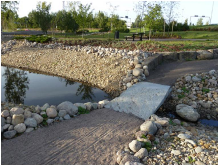
**Figure 14.** Cheek stones from a local stone processing factory are applied as bridges in the Saunaranannpuisto Park. Photo: Hannu Tolonen.
