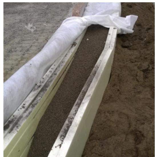
Figure 4. Frost protection of cheek stone slabs. Photo: Miikael Tolonen.
