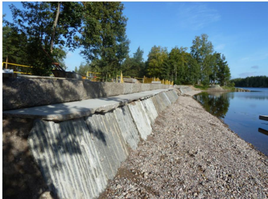
Blocks of leftover stone and cheek stones are applied in the construction of an embankment in the Myllysaaren perhepuisto Park in Lappeenranta. Photo: Hannu Tolonen.
