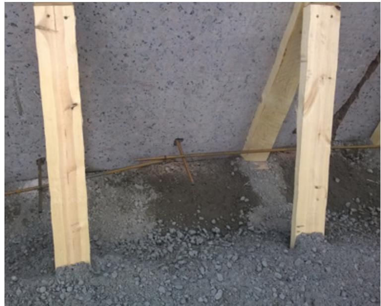
Figure 2. Reinforcement of cheek stone slabs. Photo: Miikael Tolonen.
