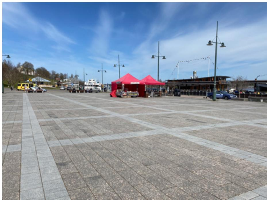
**Figure 9.** The Satamatori Square at the Lappeenranta Harbour is paved with slabs of brown rapakivi granite of Ylämaa (*Baltic Brown*) and grey granite from Kuru (*Kuru Grey*). Photo: Olavi Selonen.
