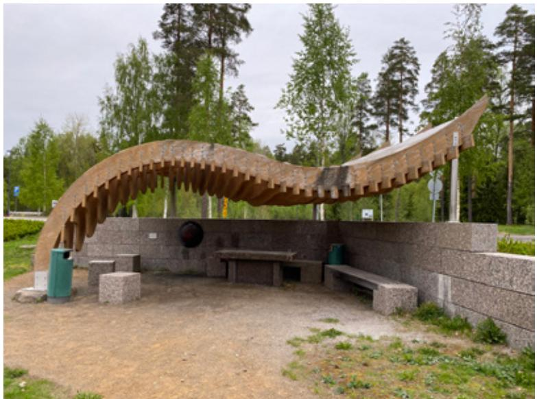
**Figure 11.** The brown rapakivi granite from Ylämaa (*Baltic Brown*) is applied as walls, stairs, benches, table, and bench legs in the outdoor recreational space of the LAB University of Applied Sciences. Photo: Olavi Selonen.
