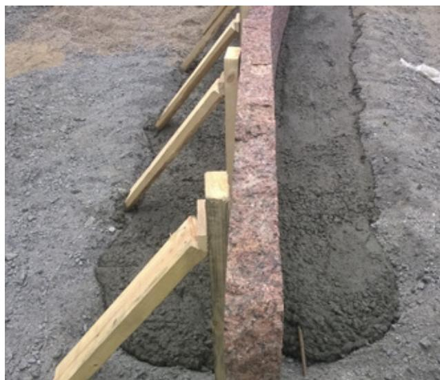
Figure 3. Casting of cheek stone slabs. Photo: Miikael Tolonen.
