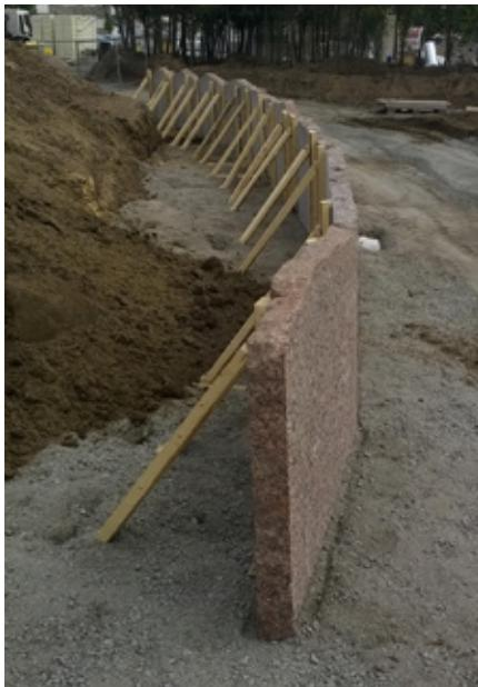
Figure 1. Cheek stone slabs leaning against the wooden stands. Photo: Miikael Tolonen.
