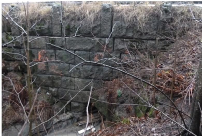
A bridge built of natural stone on the Läntinen Kanavatie Street in Lappeenranta. The bridge was demolished in connection with street construction work. The stones of the bridge were used to make a new bridge in the Saunaranannanpuisto Park (Cover Photo). Photo: Hannu Tolonen.
