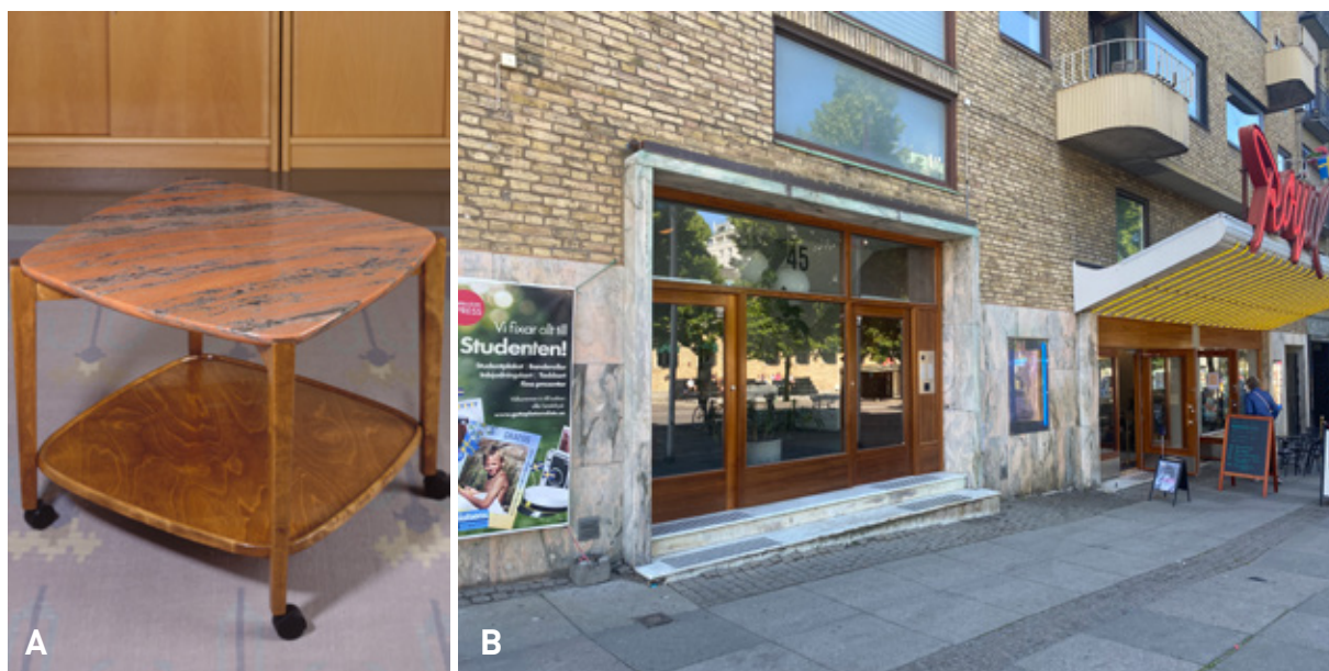
Figure 3. Objects in Nordsjö marble. A. Table top. B. Lower façade and portals (1940). No. 45 Kungsporsavenyen Street, Göteborg, Sweden. Photo A: Jari Väättäinen, Geological Survey of Finland, GTK, B: Olavi Selonen.
