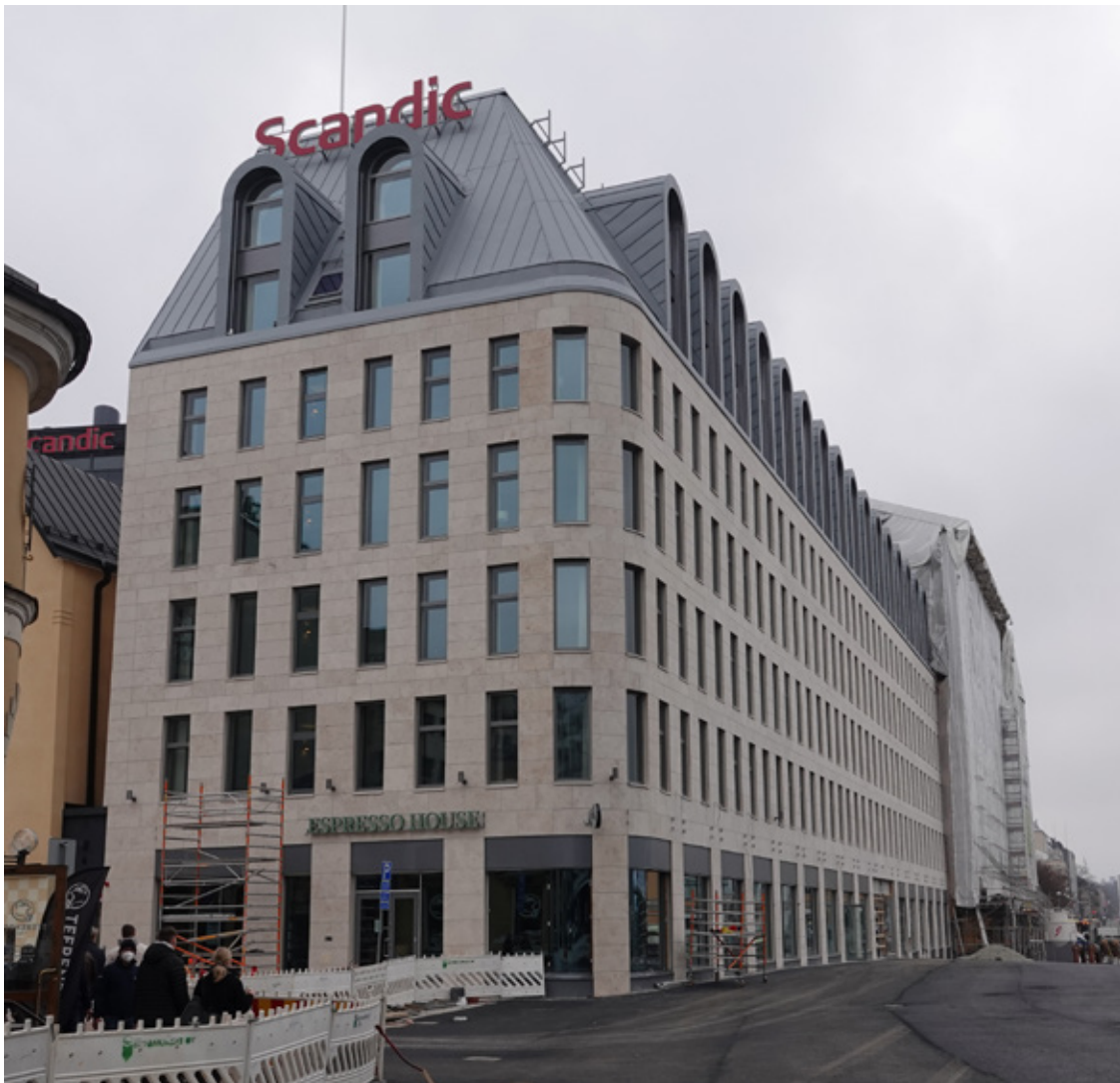
Figure 17. The New Hamburger Börs Hotel building is faced with slabs of light-coloured beige Jura limestone from Germany. Ammonite fossils can be seen on the walls. Photo: Carl Ehlers.
