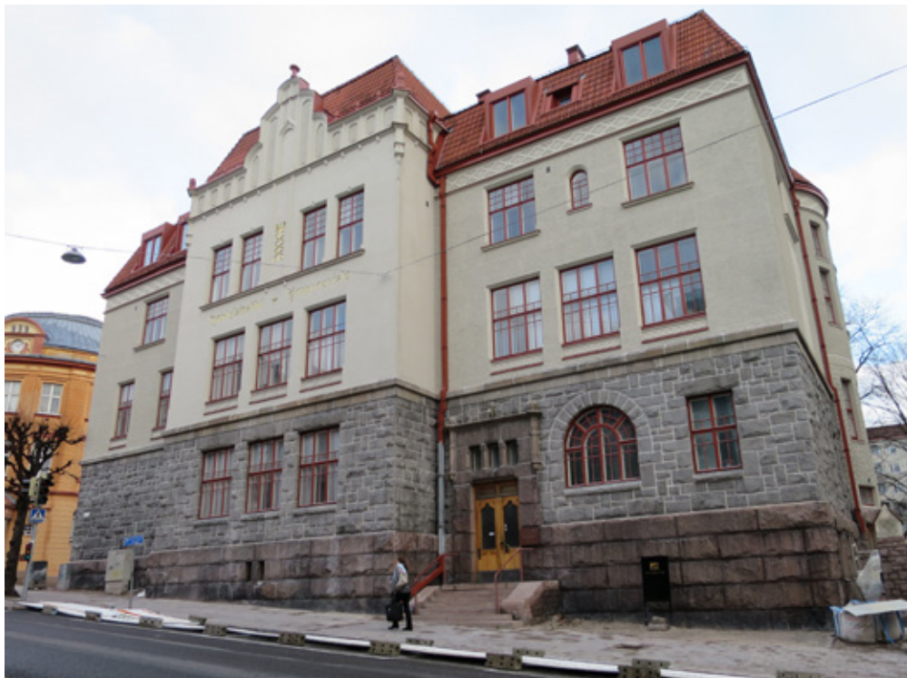
Figure 8. The foundation, portal, and stairs of the Turku School of Commerce building are composed of local rock-faced and pointed red granite from Turku. The lower façade is made of rock-faced grey granite (trondhemite) ( Birkhall Grey/Glencoe Grey ) from Uusikaupunki. Photo: Olavi Selonen.
