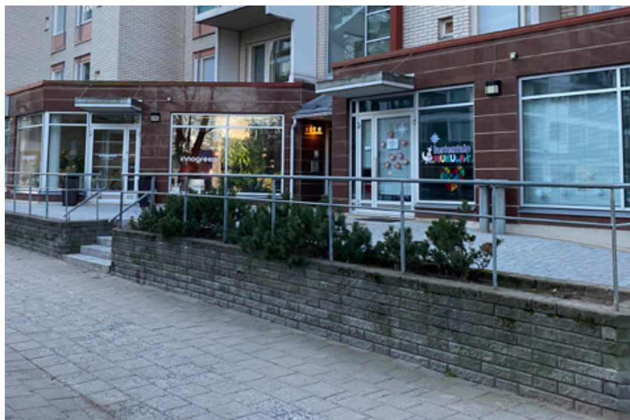
Figure 20. The lower façade of the office and apartment house at No 18 Käsityöläiskatu Street, is covered with polished slabs of red rapakivi granite from Vehmaa ( Balmoral Red fg ). Photo: Olavi Selonen.
