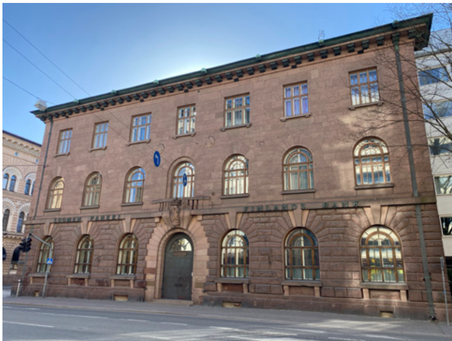
Figure 10. The façade of the Bank of Finland building is made of massive rock-faced and pointed red granite from Hanko. Photo: Olavi Selonen.
