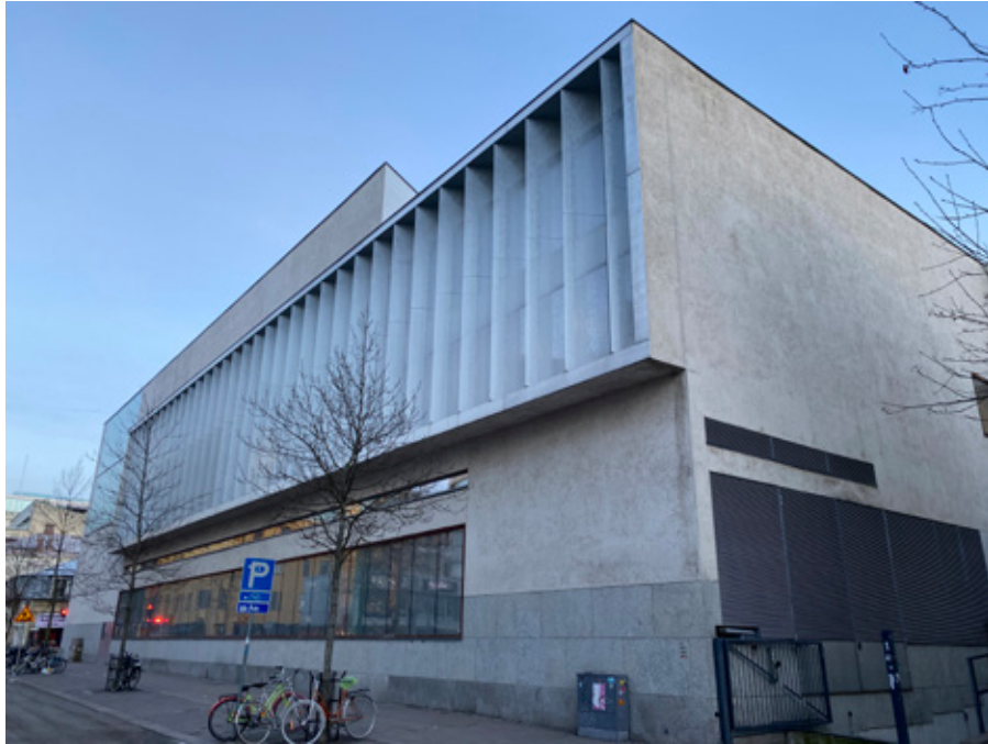
Figure 22. The lower façade of the New City Library building is clad with bush hammered slabs of yellowish granite (monzo-granite) from Viitasaari ( Viitasaari Light ). Photo: Olavi Selonen.
