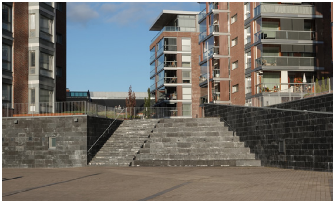
Figure 23. Slabs of Chinese schist is applied in the lower façades, walls, plinths, and stairs of the houses at the Telakkaranta apartment area by the Aurajoki River. Photo: Carl Ehlers.
