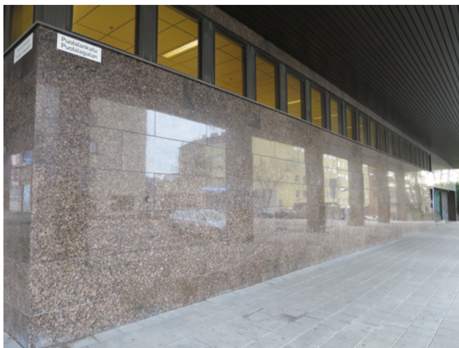
Figure 18. The lower façade of the office building at No 5 Puolalankatu Street is covered with polished slabs of brown rapakivi granite from Ylämaa ( Baltic Brown ). The traditional texture of rapakivi granite with large round K-feldspar megacrysts (ovoids), surrounded by a plagioclase mantle is well-exposed here. Photo: Olavi Selonen.
