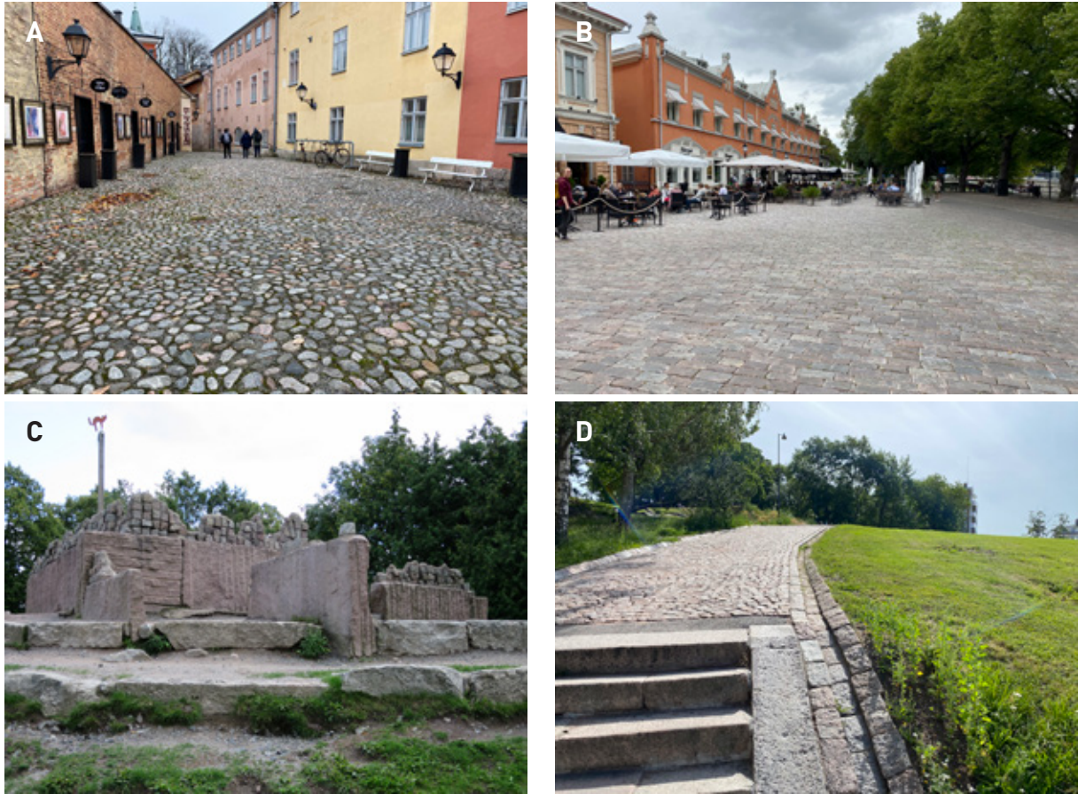
Figure 24. A. Cobble stone paving inside the Old Great Square. B. The Vähätori Square was paved with recycled sett stones made of local granites from Turku during 2009, and the pedestrian zones were covered with shot blasted small slabs of red granite from Lieto ( Lieto Red ). C. The Stone Castle, at the Adventure Park Seikkailupuisto, constructed of leftover stone from one of the Balmoral Red cg quarries represents a good example of use of the leftover. D. Natural stone applied as stairs, kerbs, and paving at the Puolalanpuisto Park. Photos: Olavi Selonen.
