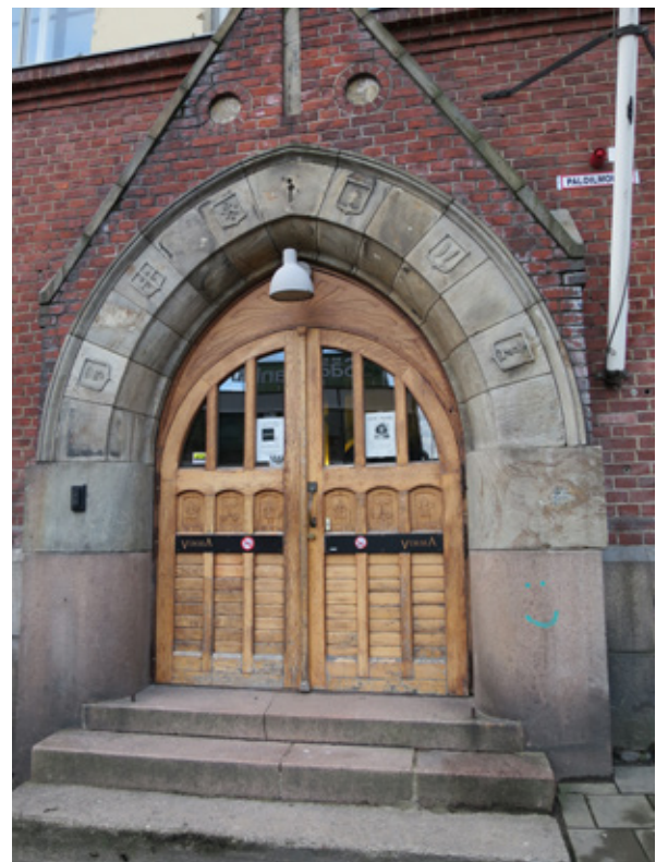
Figure 6. The ornate portal of the Girls' school building is composed of Finnish soapstone from Nunnanlahti. Photo: Olavi Selonen.
