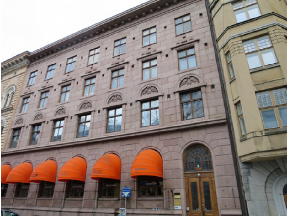
Figure 9. The façade of the extension to the Savings Bank building is covered with pointed red rapakivi granite from Taivassalo ( Balmoral Red cg ). Photo: Olavi Selonen.
