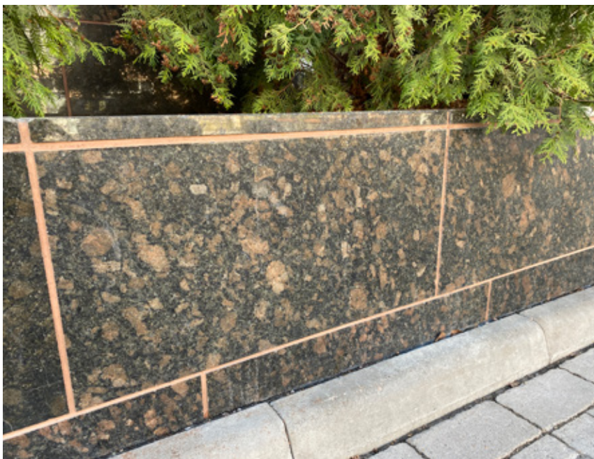
Figure 5. The plinth of the Patria hotel building is clad with reddish brown porphyritic granite (granodiorite) from the village of Korkea-aho ( Finlandia Brown/Karelia Rosa ). Photo: Olavi Selonen.
