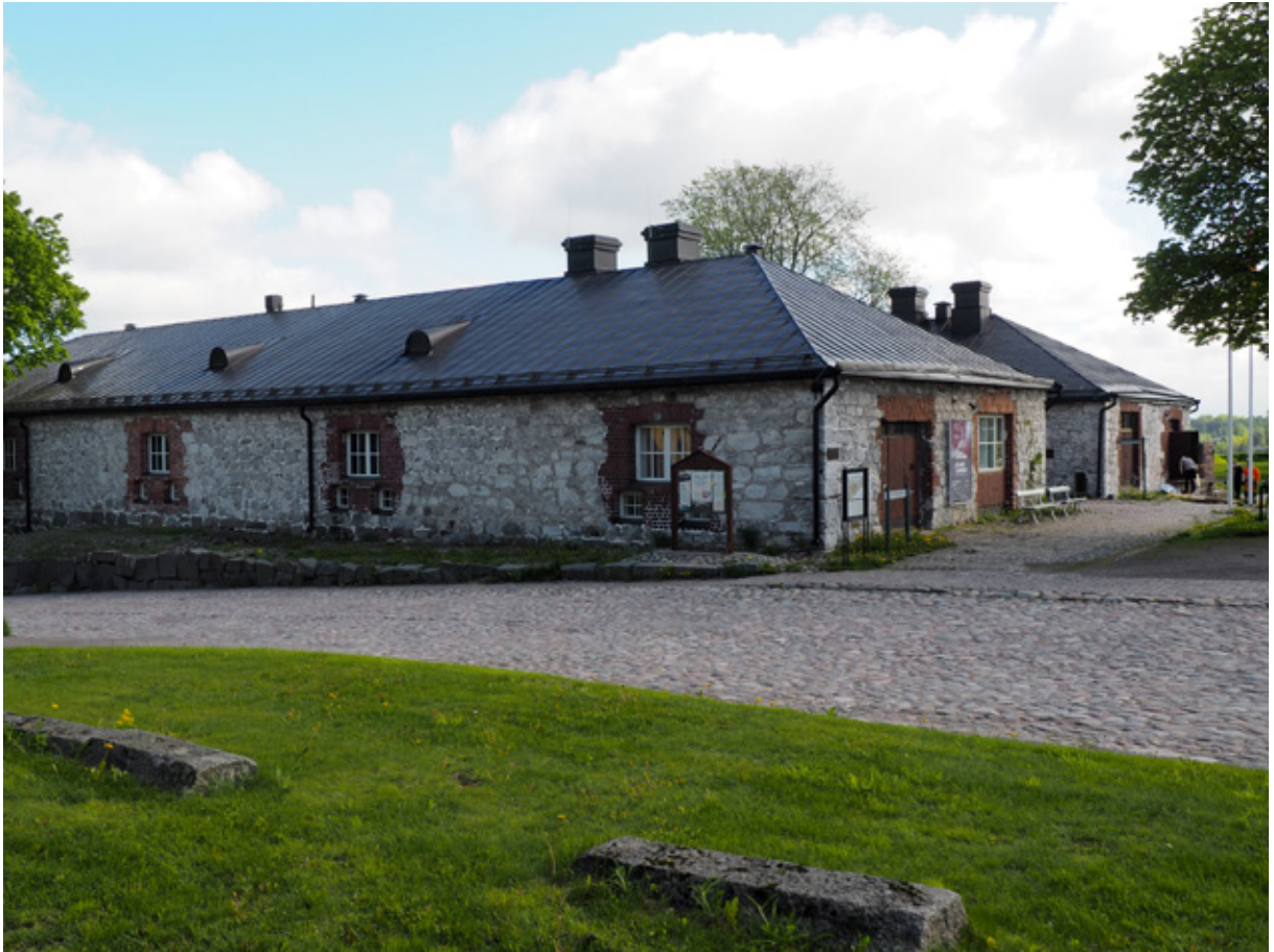
Figure 2. The South Karelia Museum. Blocks of local hard granitic rock types are applied in the lower parts of the buildings and blocks of limestone from the local Ihalainen quarry in the upper parts. Photo: Heidi Laxström.
