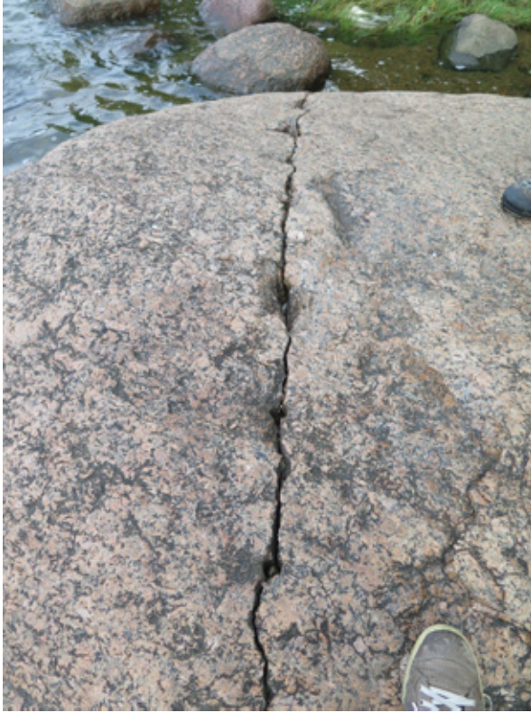
Figure 2. Stones for the churches designed by Josef Stenbäck were always quarried locally. The picture shows traces of cleaved rapakivi granite at a distance of approx. 50 m from the Koivisto church. Photo: Heikki Pirinen.
