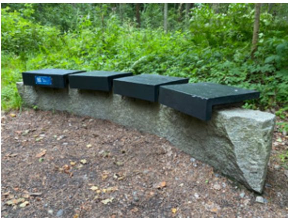
Figure 6. The pedestal of the bench in the Lanu-puisto Park is made in grey granite from Kuru (Kuru Grey). Photo: Olavi Selonen.
