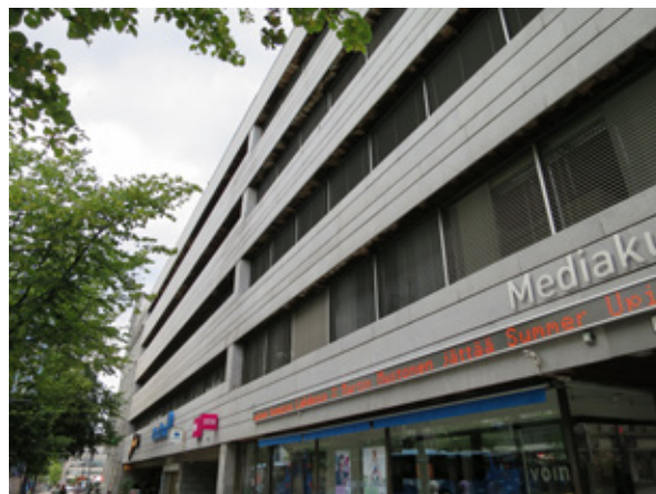
Figure 2. The façade of the extension to the Lahti KOP bank building is faced with grey Uusikaupunki granite (trondhjemitte) (Birkhall Grey/Glencoe Grey). Photo: Olavi Selonen.
