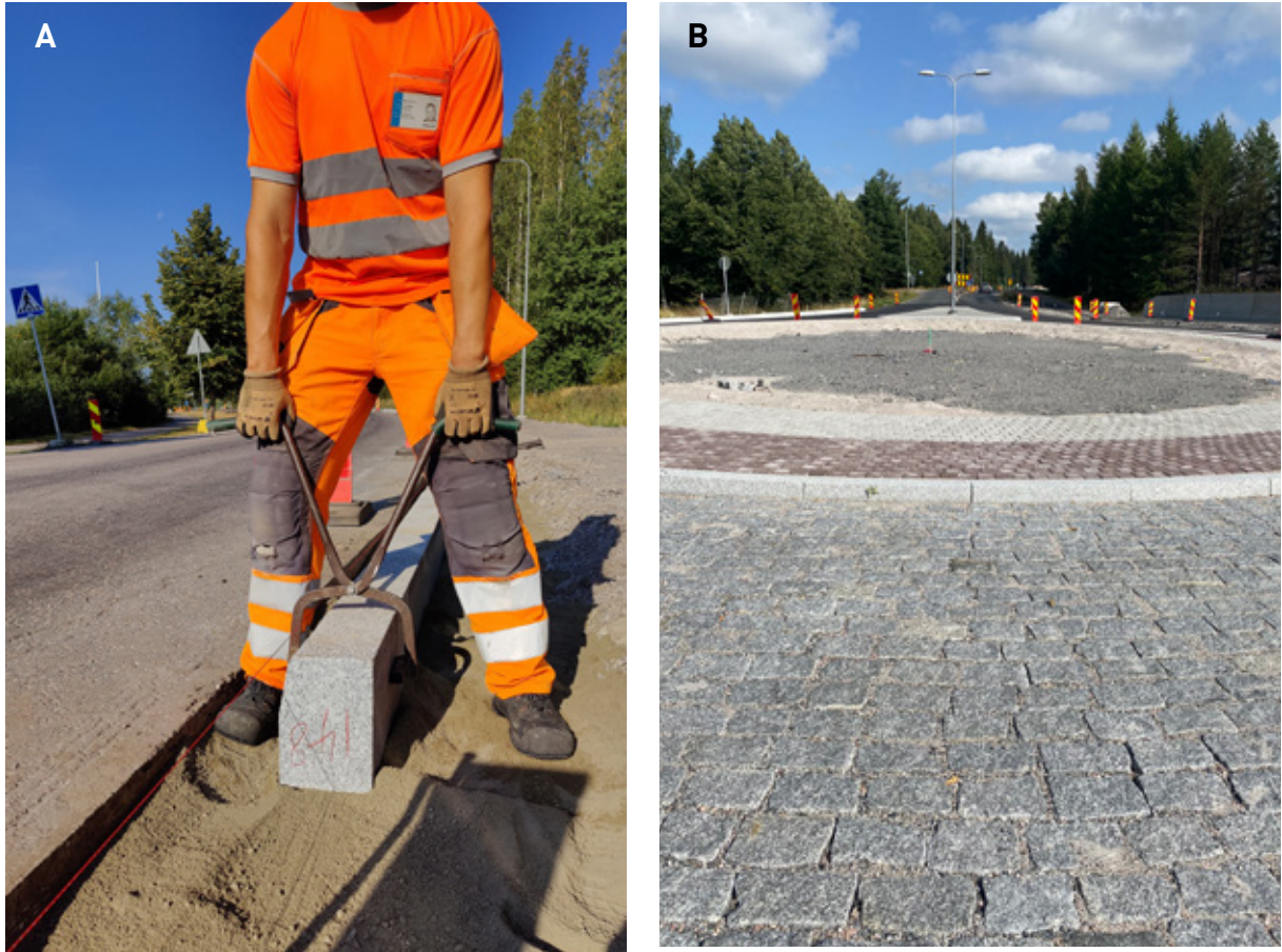
Figure 8. A. Installation of kerbstones along the Helsingintie Street in 2022. B. Roundabout at the Helsingintie Street in 2022. The grey granite from Ristijärvi ( Ristijärvi Grey ) is applied. Photos A: Sini Laine, B: Olavi Selonen.
