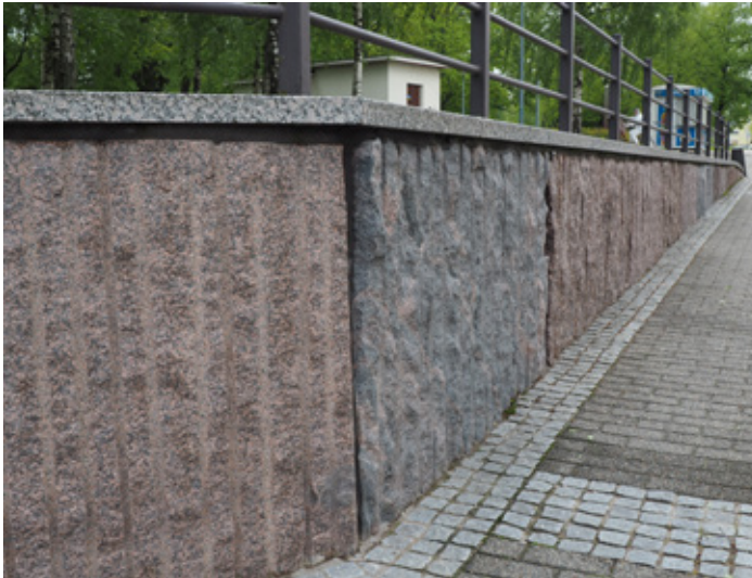
Figure 10. The natural stone wall at the Kauppakatu Street is made of leftover stone from a local stone processing factory. The wall consists of multi-coloured granite (migmatite) from Sulkava ( Amadeus ), red-black granite (migmatite) from Mäntsälä ( Aurora ), red rapakivi granite from Taivassalo ( Balmoral Red cg ) and red rapakivi granite from Virolahti ( Carmen Red ). Photo: Heidi Laxström.
