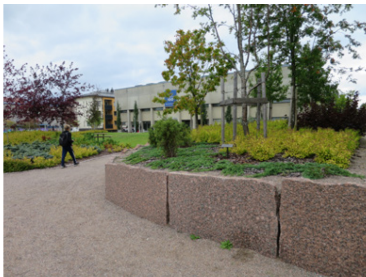
Figure 12. Cheek stones from a local stone processing factory are applied as walls in the Paasikivenpuisto Park. The surface has a flamed finish. Photo: Olavi Selonen.
