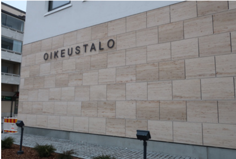
Figure 7. Lappeenranta Court House. The lower façade of the building is clad with Jura limestone from Germany. Photo: Paavo Härmä.
