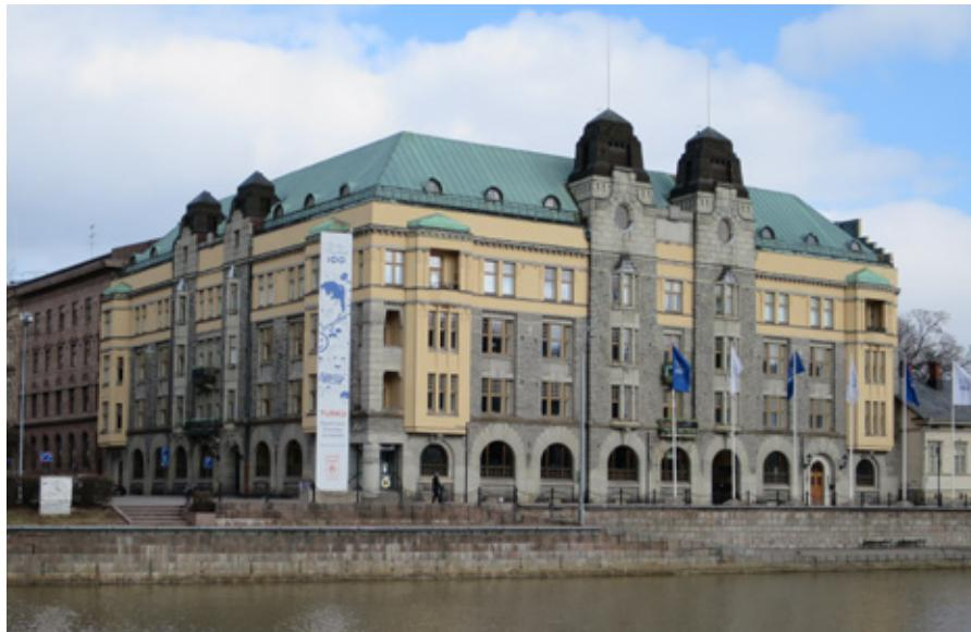
**Figure 7.** The façade of the Fire Insurance Company building is partly made of rock-faced and pointed light grey granite (trondhjemite) from Uusikaupunki (*Birkhall Grey/Glencoe Grey*). Photo: Olavi Selonen.
