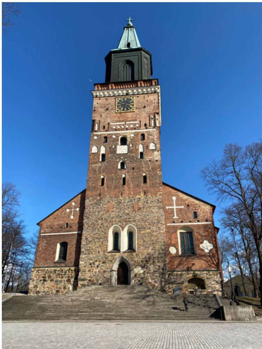
**Figure 2.** A mixture of local rock types of varying shapes are used in construction of the foundation of the Turku Cathedral. Photo: Olavi Selonen.
