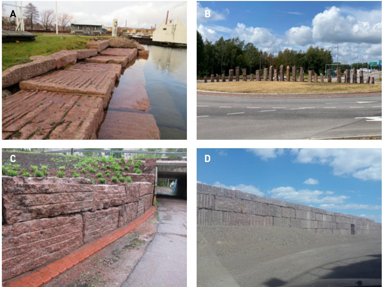
**Figure 14.** Applications made of leftover stone in the City of Kotka. A. Embankment in Meriniemi by the Guest Harbour. B. Columns at the Uittoväylä roundabout in the Jumalniemi suburb. C. Masonry in Karhuvuori. D. 120-metre long granite wall in the Mussalo Harbour. Photos A, B: Olavi Selonen, C: Paavo Härmä. D: Linjaporaus Lehtinen Oy.
