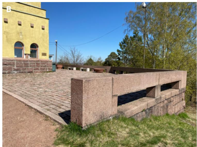
**Figure 4.** The Haukkavuori Observation Tower is situated at No 51 Keskuskatu Street (A). The plinth, masonry, stairs, yard paving, and decorations of the Tower are made of local red rapakivi granite from Metsola (B). Photos: Olavi Selonen.
