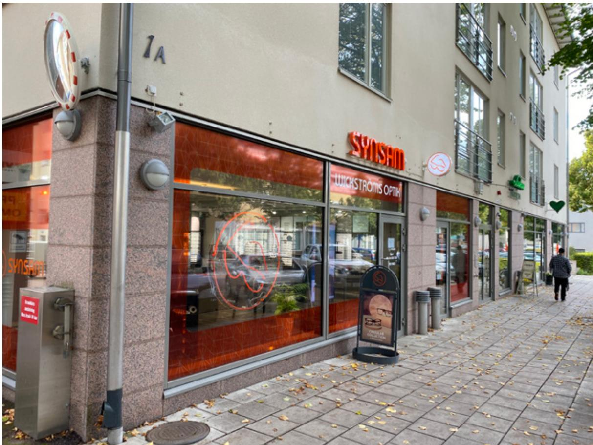
**Figure 17.** The lower façade of the building at No 1A Norragatan Street in Mariehamn is faced with slabs of *Balmoral Red* cg granite. Photo: Olavi Selonen.
