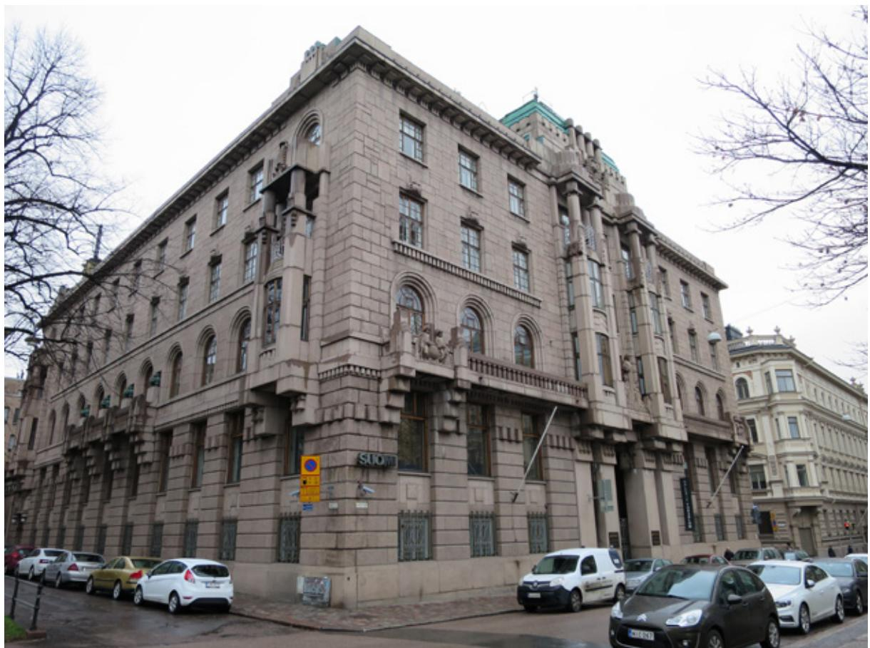
**Figure 3.** The façade of the building of the Insurance Company Suomi in Helsinki is made of pointed Kökar granite.
