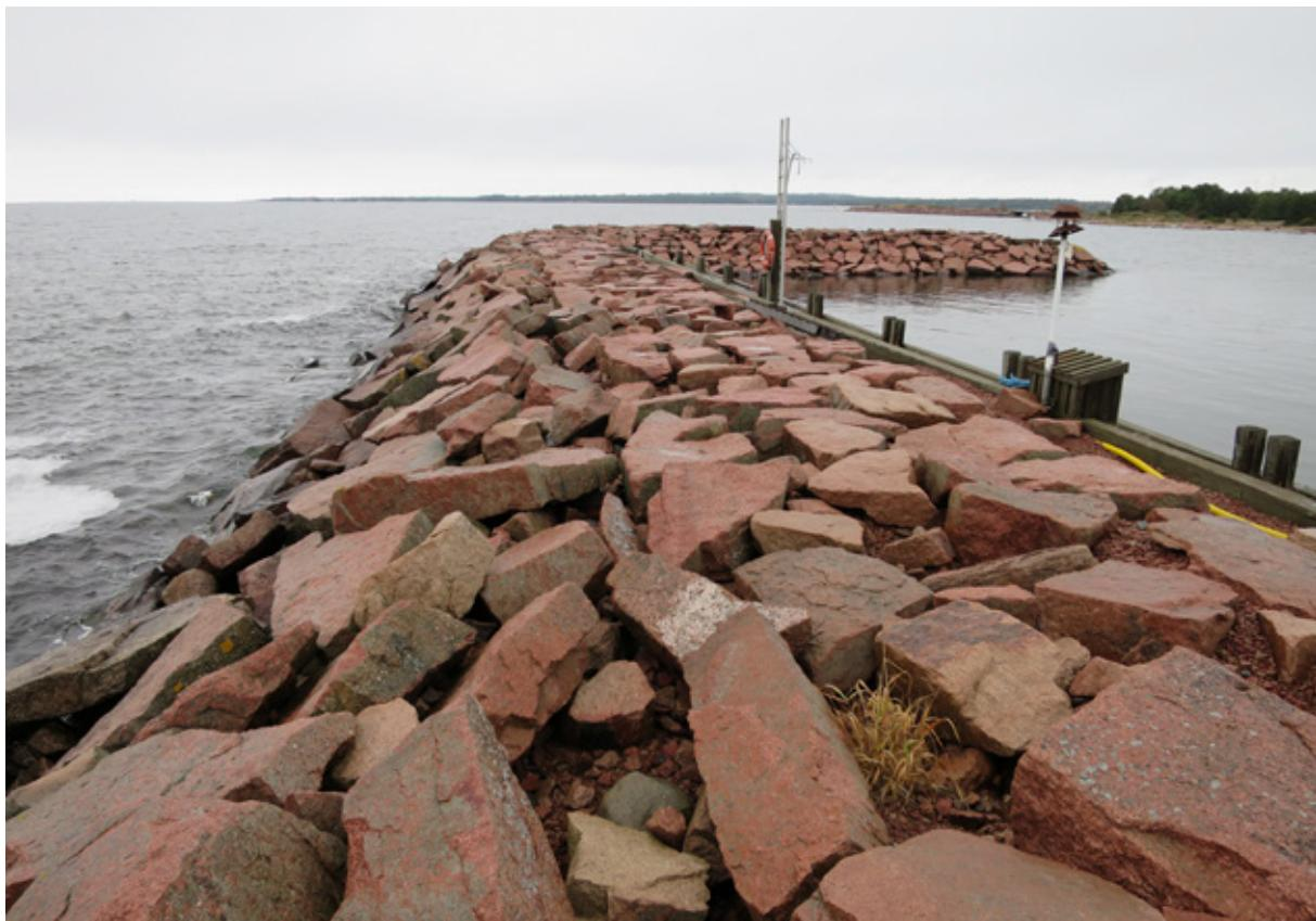
**Figure 24.** The breakwater by the Eckerö Post Bridge comprises mostly armourstone blocks of local red rapakivi granite. Photo: Olavi Selonen.
