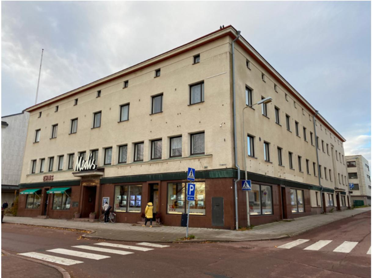
**Figure 16.** The lower façade of the building at No 1 Styrmansgatan Street in Mariehamn is made of slabs of *Balmoral Red fg* granite. Photo: Olavi Selonen.
