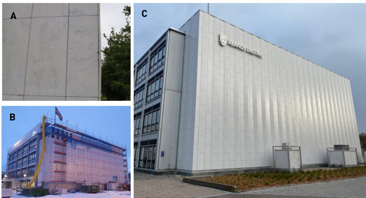
**Figure 15.** The façade of the Self-government House in Mariehamn was originally made of slabs of Carrara Marble. Due to fluctuations of air temperature and humidity, the slabs bended (A), and were replaced during 2020–21 (B) with slabs of glazed terracotta from Germany. (C) Final façade in 2021. Photos: A, C: Olavi Selonen, B: Daniel Andersson.
