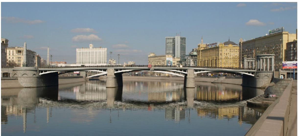
**Figure 5.** Stone supports, obelisk, and columns in the Borodino Bridge in Moscow are made in grey Kumlinge granite in 1915. Source: [https://commons.wikimedia.org/wiki/File:Moscow,\\_Borodinsky\\_Bridge\\_02.jpg](https://commons.wikimedia.org/wiki/File:Moscow,_Borodinsky_Bridge_02.jpg).
