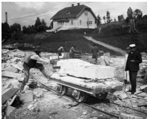
Figure 7. Processing of soapstone at the beginning of the 1900's was done either by hand or by mechanized saws (Kotivuori 1981). The handsaws were double-handed saws that later were substituted by one-handed saws. Motorized saws in the factories included gang saws and circular saws. Soapstone plant in Nunnanlahti, Juuka. Photo: W.W. Wilkman, summer 1909. GTK, Old pictures no 5891.
