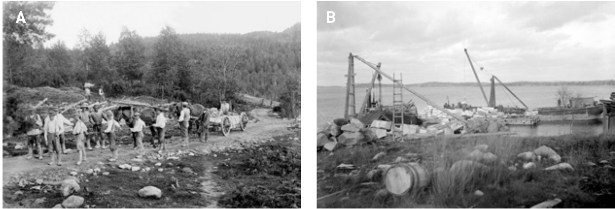
Figure 8. At the early 20 th century, transport of stone in the Mustavaara quarry was done by horse pulled mine carts (A); and from the quarry to harbour with horse pulled carts on rails. Soapstones were transported from the Nunnanlahti harbour by boats (B) to the cities of Helsinki, Vyborg, and Saint Petersburg. During wintertime (if necessary), the stones were transported on ice by horse pulled sledges, e.g. to the city of Joensuu. Later, from the 1910's, (after the expansion of the railroad network) transport of stone by train to Helsinki and Vyborg became an option. Photos: A. Benjamin Frosterus, 1904. GTK, Old pictures no 1208. B. Benjamin Frosterus, 1904. GTK, Old pictures no 1205.
