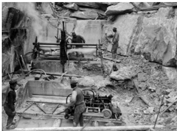
Figure 6. In the early 1900's, soapstone was loosened from the bedrock by piston drills and later by hammer drills (Kotivuori 1981). Vertical and horizontal holes were drilled next to each other and channelling was done with the same drills. Power was initially provided by steam, and from the middle of the 1910's the steam power was gradually replaced by compressed air. Large cranes were used for lifting stone blocks in the quarry. Mustavaara quarry in Nunnanlahti, Juuka. Photo: Benjamin Frosterus, 1904. GTK, Old pictures no 1213a.
