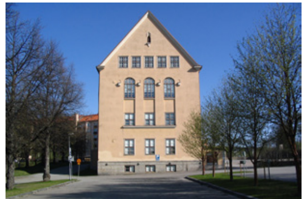
Figure 10. The south gable of the Niirala School building. Photo: Heikki Lukkarinen.
