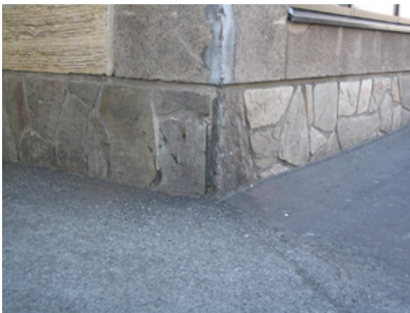
Figure 25. Quartzite tiles on a plinth. Photo: Heikki Lukkarinen.
