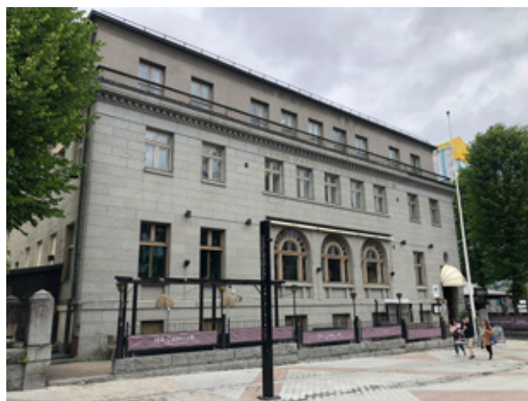
Figure 8. The Bank of Finland. Photo: Olavi Selonen.
