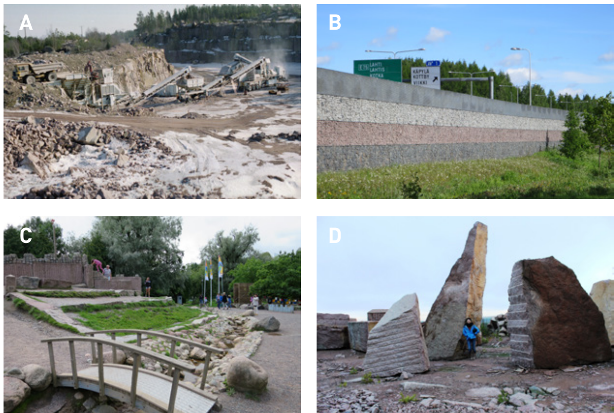
Figure 19. Use of leftover stone in the Vehmaa batholith. A. Crushing of the leftover of the Vehmaa granite. Photo: Olavi Selonen. B. Gabion as noise barrier. The third layer from the top is made of coarse aggregate of red Taivassalo granite. Photo: Olavi Selonen. C. Children's playground made of the leftover of the Taivassalo granite. Photo: Olavi Selonen. D. Monumental undressed leftover blocks of the Taivassalo granite. Photo: Reijo Leivo.
