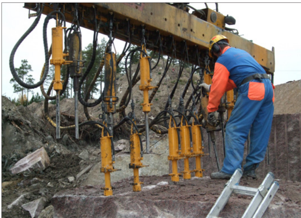
Figure 18. Hydraulic splitting of semi-finished block in the Taivassalo granite. Photo: Carl Ehlers.
