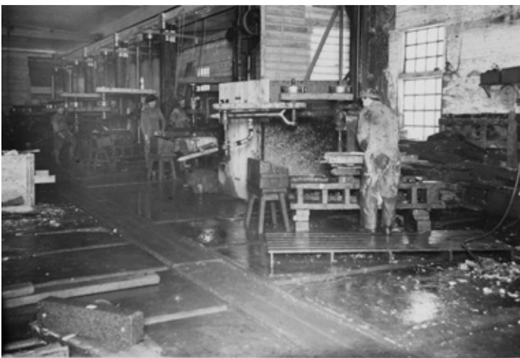
Figure 7. View of the processing plant of Ab Granit in 1936. Photo: Collection Ab Granit, The Åbo Akademi Picture Collections.
